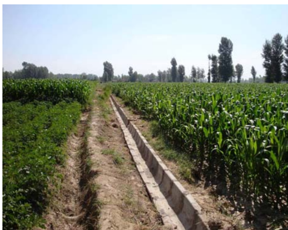
Canal lining from tubewell
