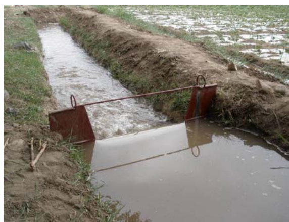
Weir in unlined channel
