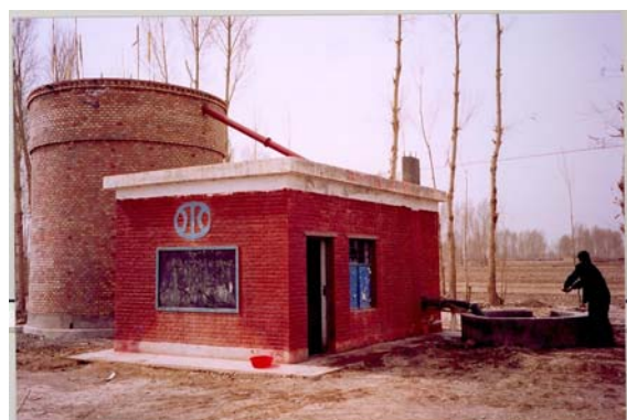
MWR pumping station
