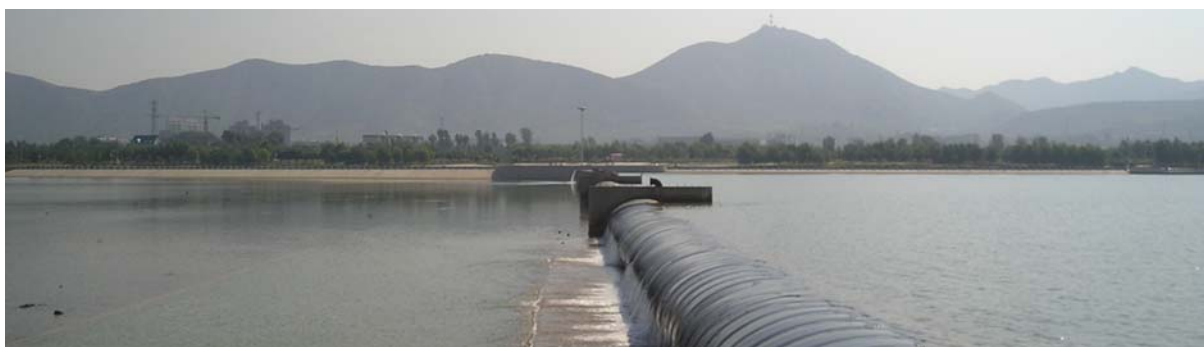
A rubber dam in Chaoyang City
