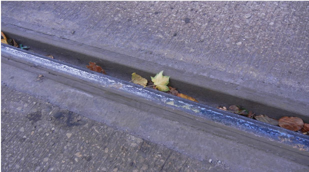
Figure 11: Photograph of rail head at Shalesmoor, taken immediately after accident. Note that rail head is black in colour and the presence of fallen leaves
