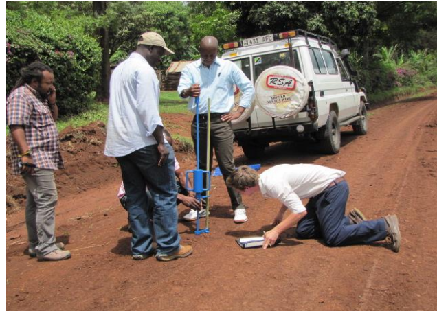
DCP measurement at Ch. 2+580
