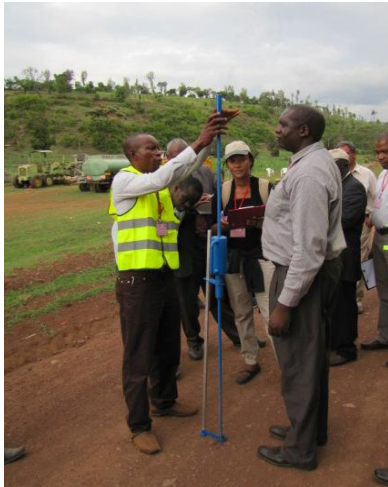
DCP measurement at Ch. 0+258
