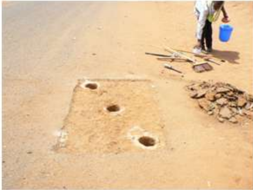
IDD testing by sand replacement method
