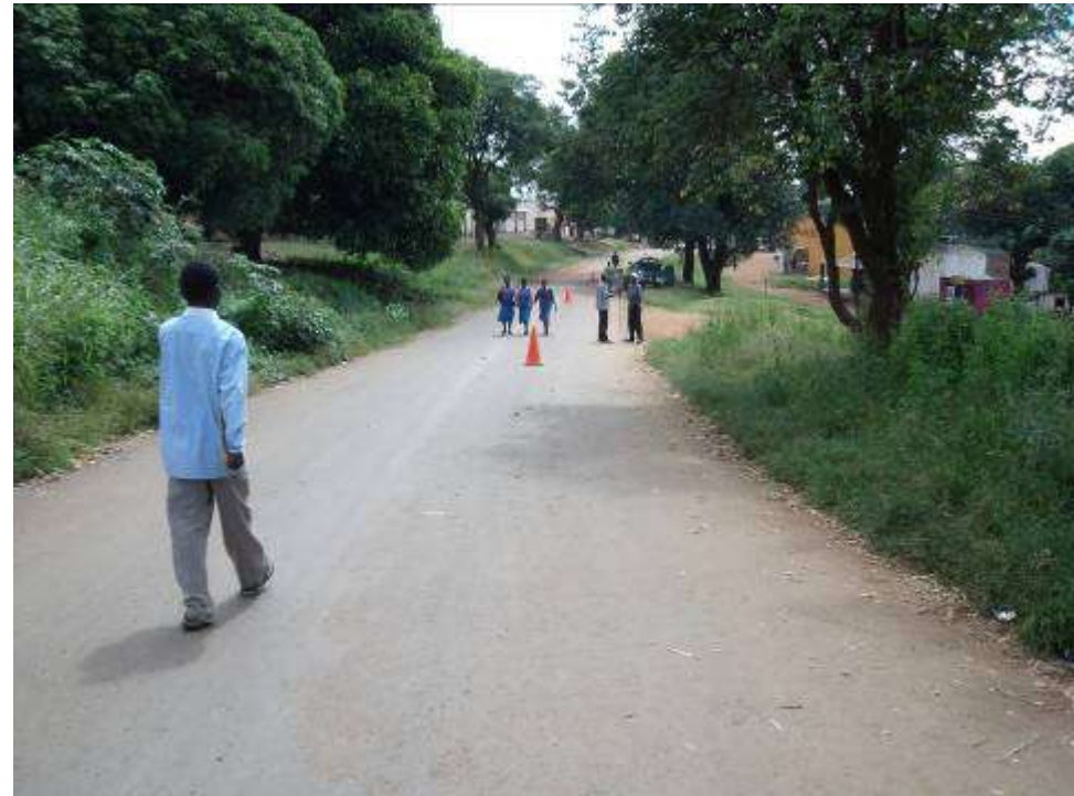
Photo: Dowa road – constructed in 2004 Condition: Good/sound
