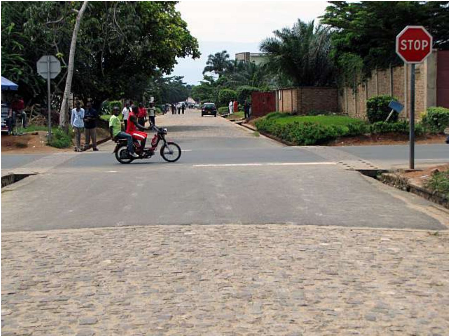
Urban road surfacing: AC on urban arterials and cobblestone on urban collectors
