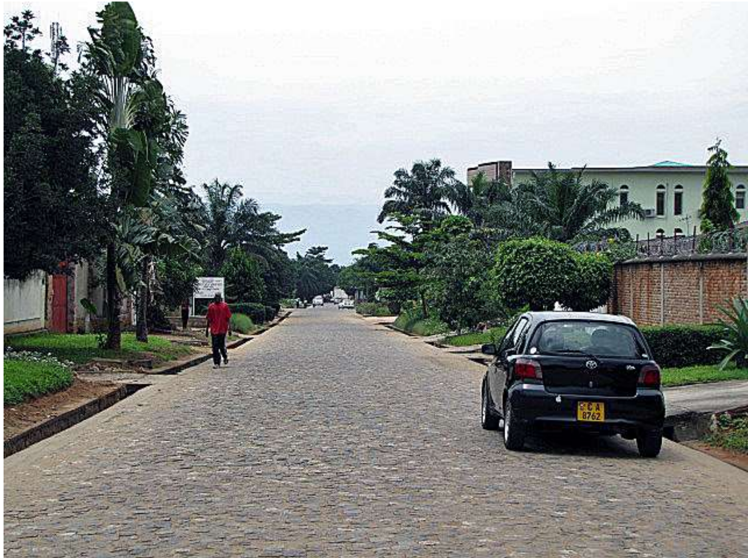
Typical cobblestone surfacing on urban collector road in Bujumbura
