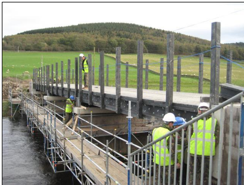
Figure 6: Longitudinal view of bridge during construction.
