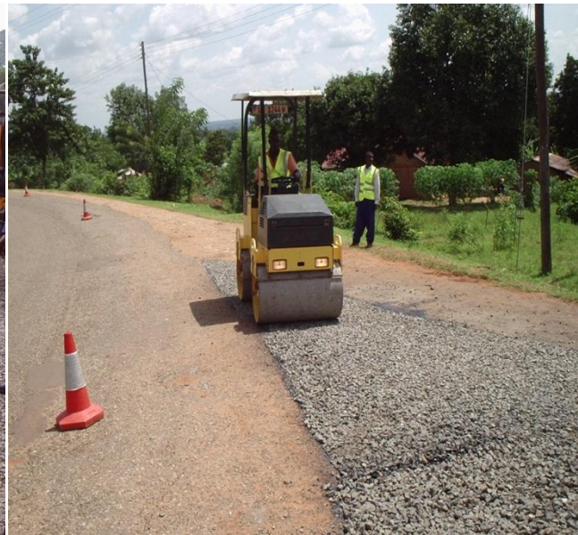
Fig-9: Rolling over 20/40 stone with 1.7 t roller
