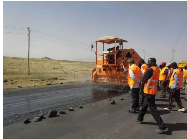
Figure 4 Chipping spreading
