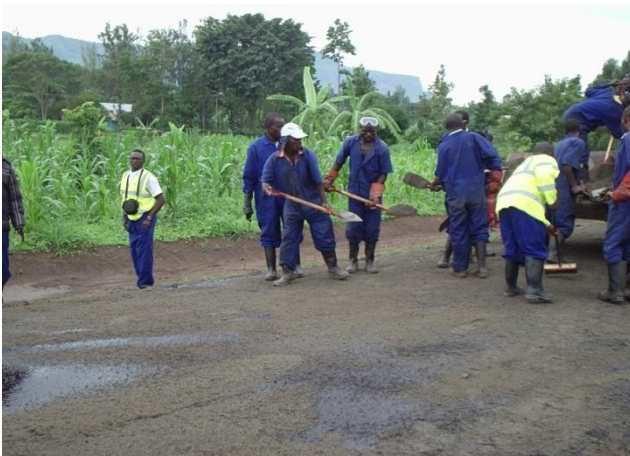
Fig-12: Quarry sand seal applied on tack coat
