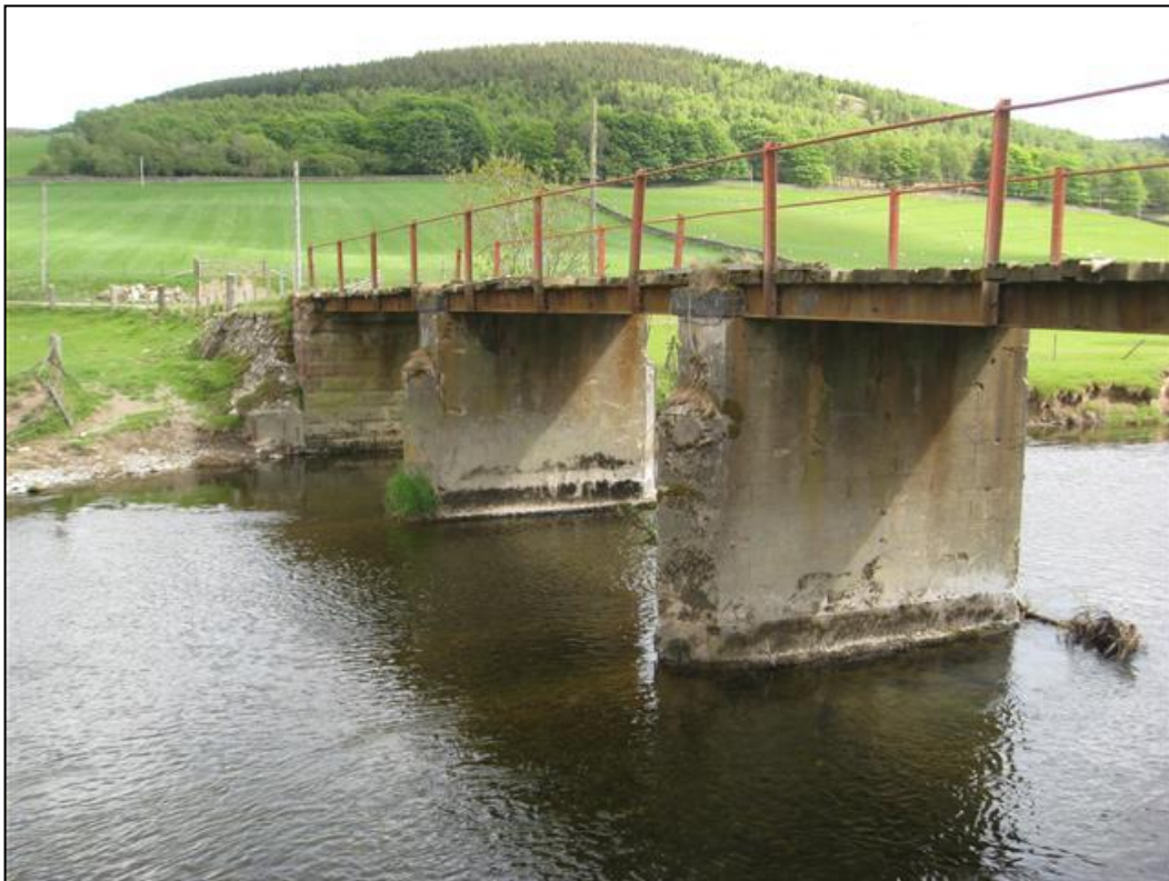
Figure 4: Dilapidated composite bridge at Easter Dawyck, Peeblesshire, Scotland.
