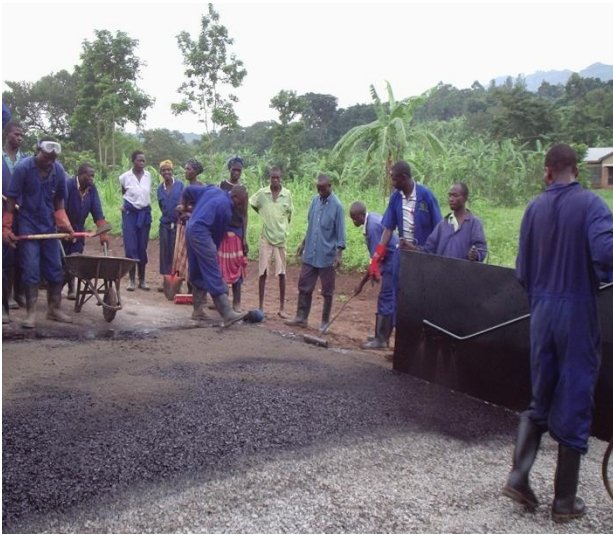
Fig-10: Applying 1.0l/m 2 on 10/14mmstone
