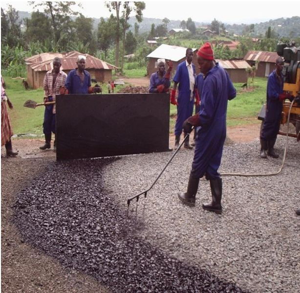
Fig-8: Applying the 2.9 l/m 2 as 1 st penetration
