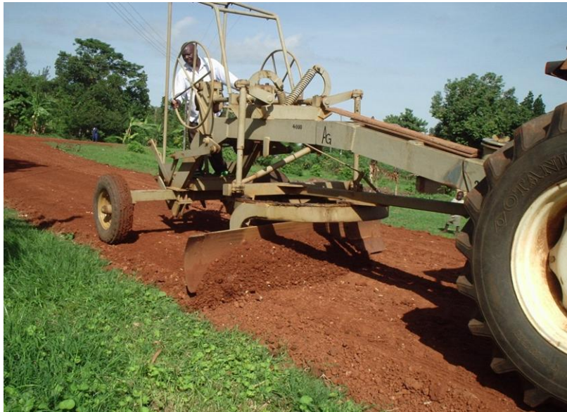
Figure-2: Busamaga – Magada final smooth cut to 3% camber using a towed grader.
