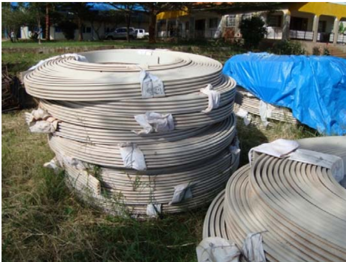
Photograph No 2 Rolls of U-PVC strips stored on site at the construction camp.
