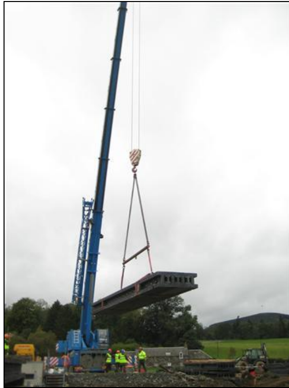
Figure 5: Typical 9 metre decking section being craned into place.
