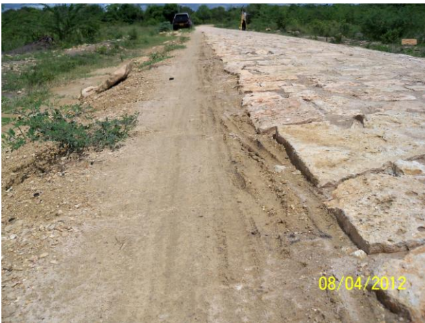
Figure 6 - Hand Packed Stone Shoulder Wear Figure 7 - Motorcycle Using Gravel Shoulder
