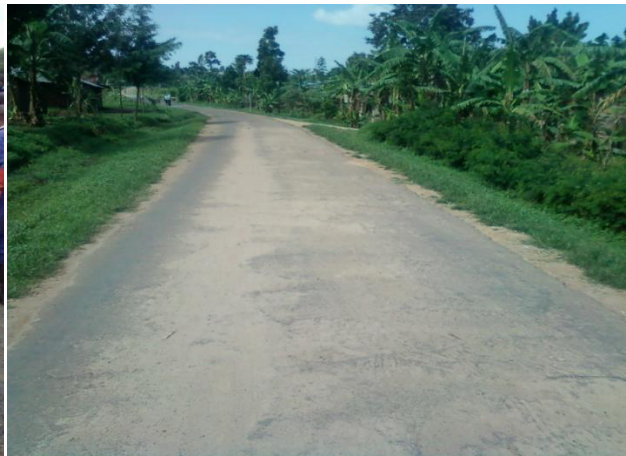
Fig-13: Completed sand seal section
