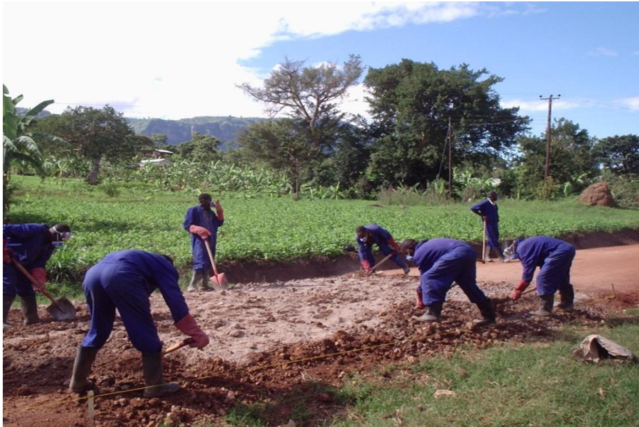
Figure-1; Base construction at Busamaga – Magada (Mbale-Uganda) with lime stabilised gravel.
