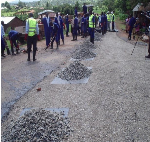
Fig-6: Spotting of 20/40mm stone
