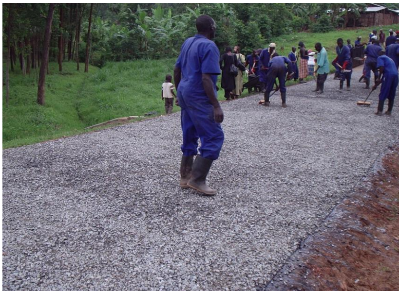
Fig-14: Single Surfaced Dressed section prior to application of fog spray
