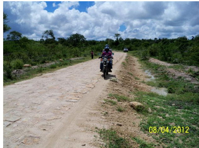
Figure 6 - Hand Packed Stone Shoulder Wear Figure 7 - Motorcycle Using Gravel Shoulder
