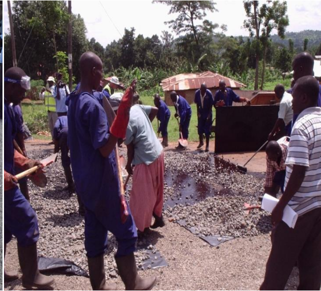
Fig-7: Laying 20/40 stone on tack coat
