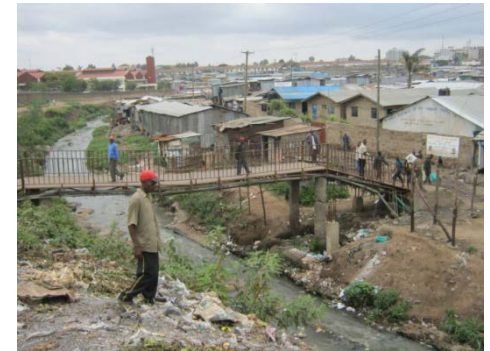
Hotspot bridge in Mukuru
