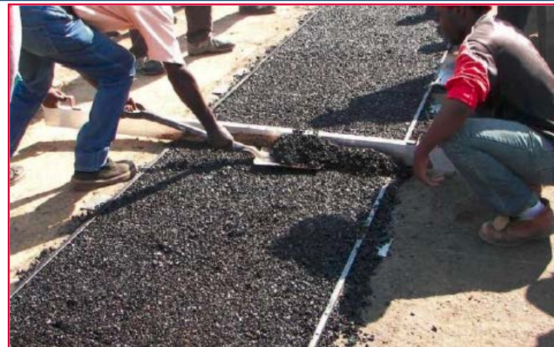
Thin cold mix asphalt
