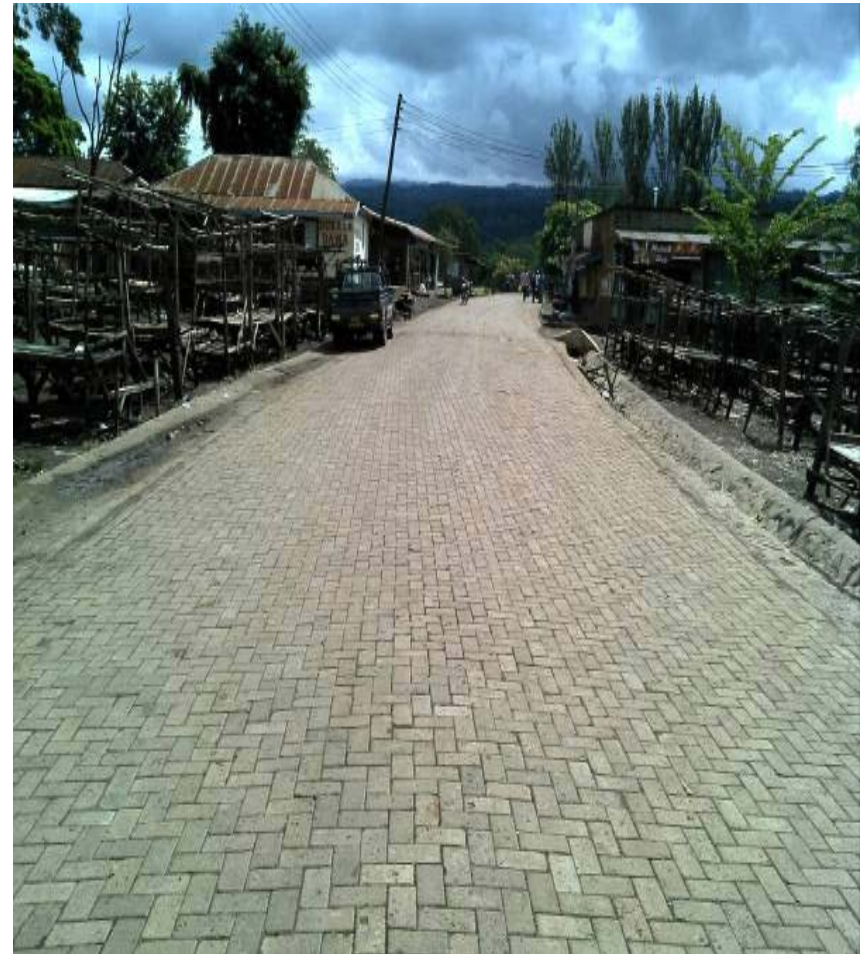
Completed Paving Block
