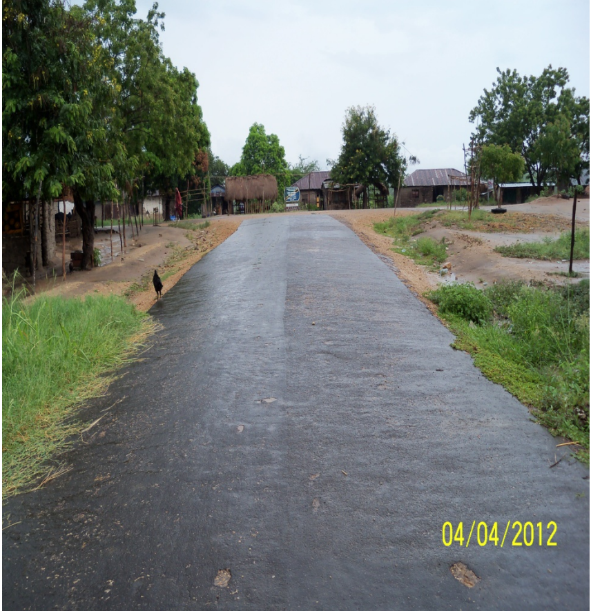
Completed Slurry Seal
