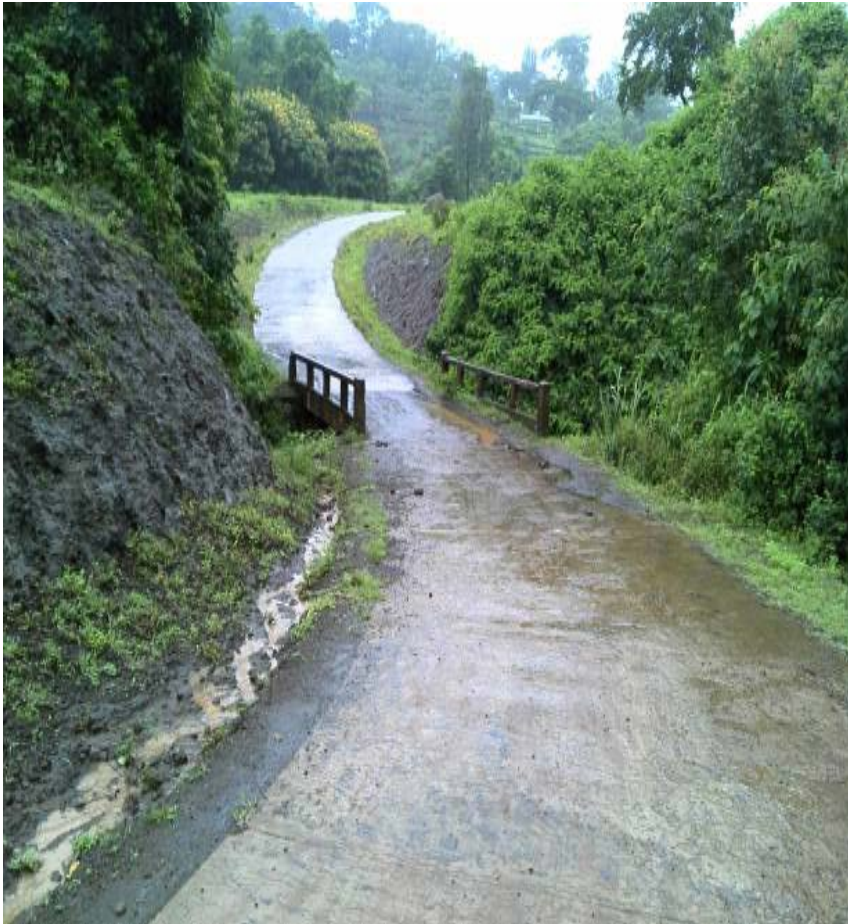
Completed Concrete Slab
