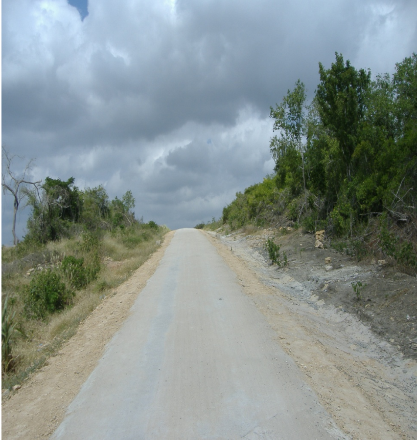
Completed Concrete Geocells
