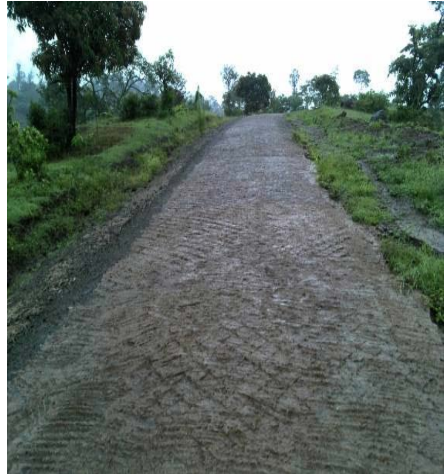
Completed Geocells Concrete
