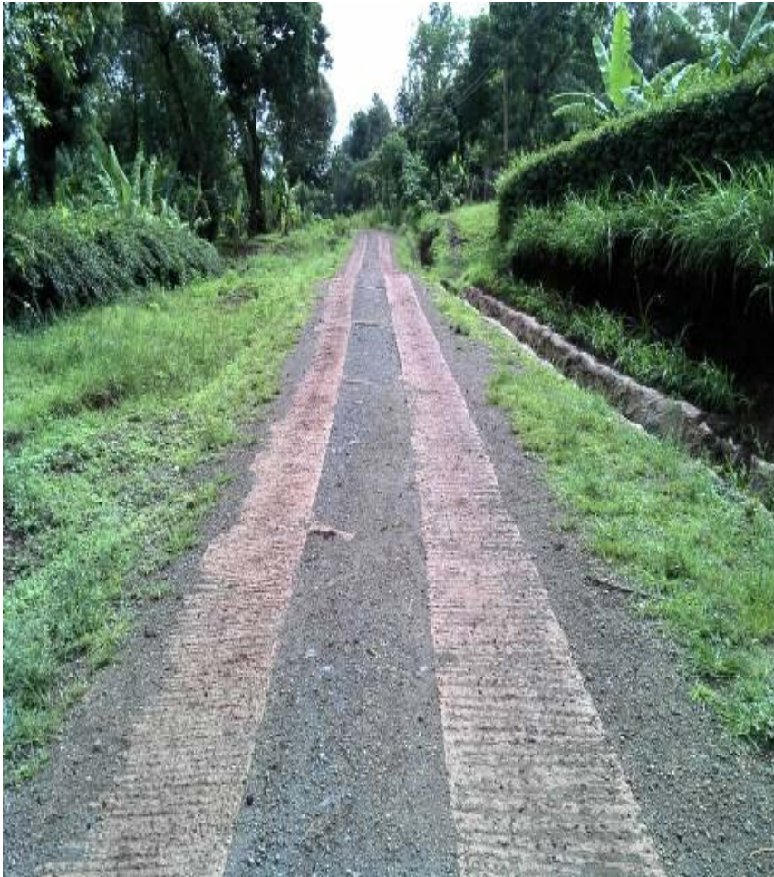
Completed Concrete Strip
