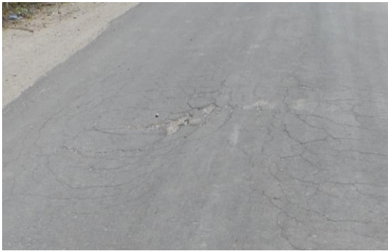
Fig. 4. Typical shear failure due to overstressing
