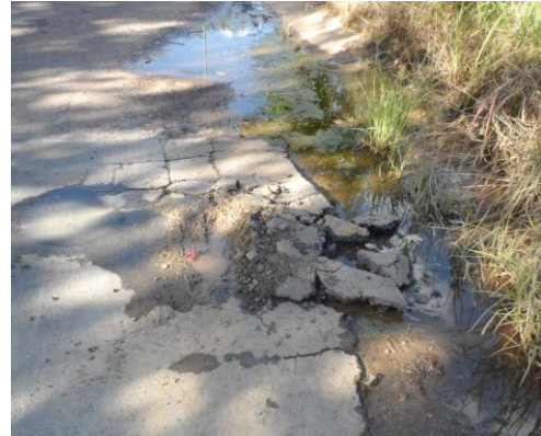
Fig. 7. Failure of a road (patch in this case) after less than 10 heavy vehicles (caused by excessive water)
