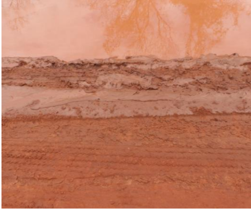
Fig. 6. Weak material (in a soaked condition) after numerous 88 kN axle passes
