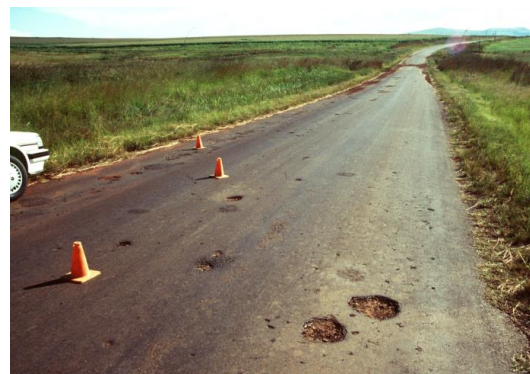
Fig. 1. Low volume road showing lack of maintenance, which ultimately leads to road failure
