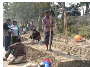
Picture-10 Field compaction test
