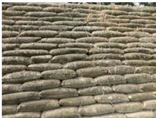
(a) Soil bag (A little deteriorated)
