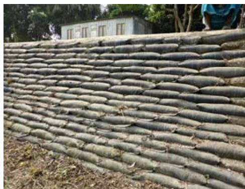
(b) Geo-synthetic bag (No deterioration)
