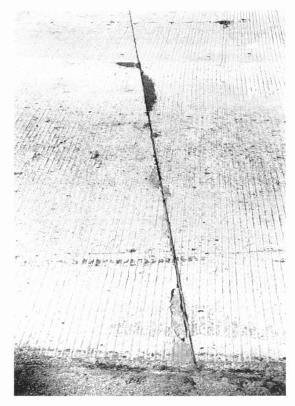
Plate 5 Spalled joint
