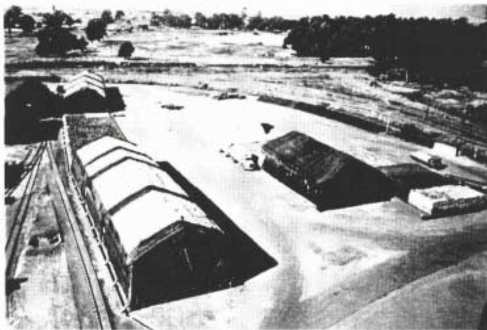
Grain Marketing Board Aspidale depot showing 4500 tonnes of maize in polypropylene bags stacked on an outdoor hardstanding in the foreground.
