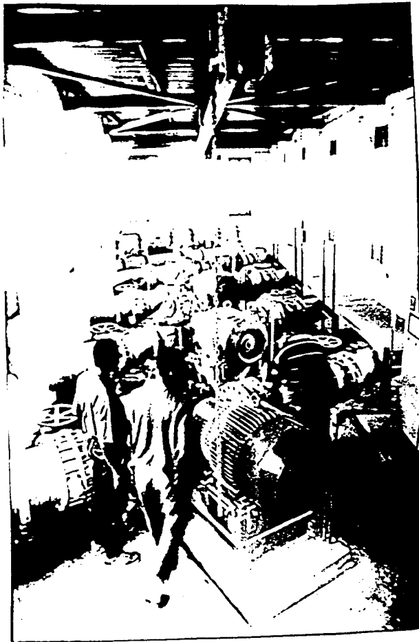
One of the 14 pump stations at Hlaneki
