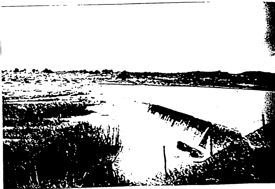
The overflow of the Piet Gouws Dam
