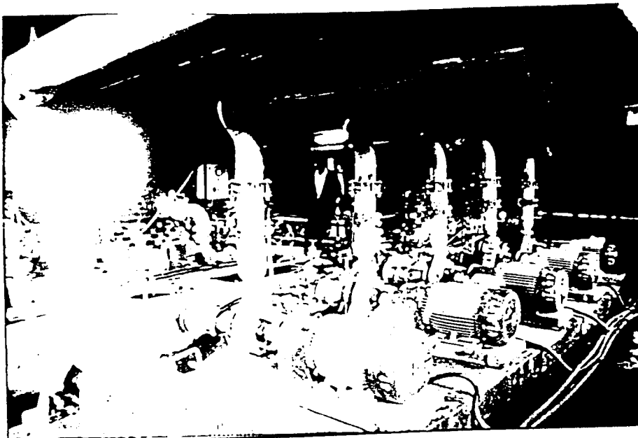
A pumpstation for sprinkler irrigation
