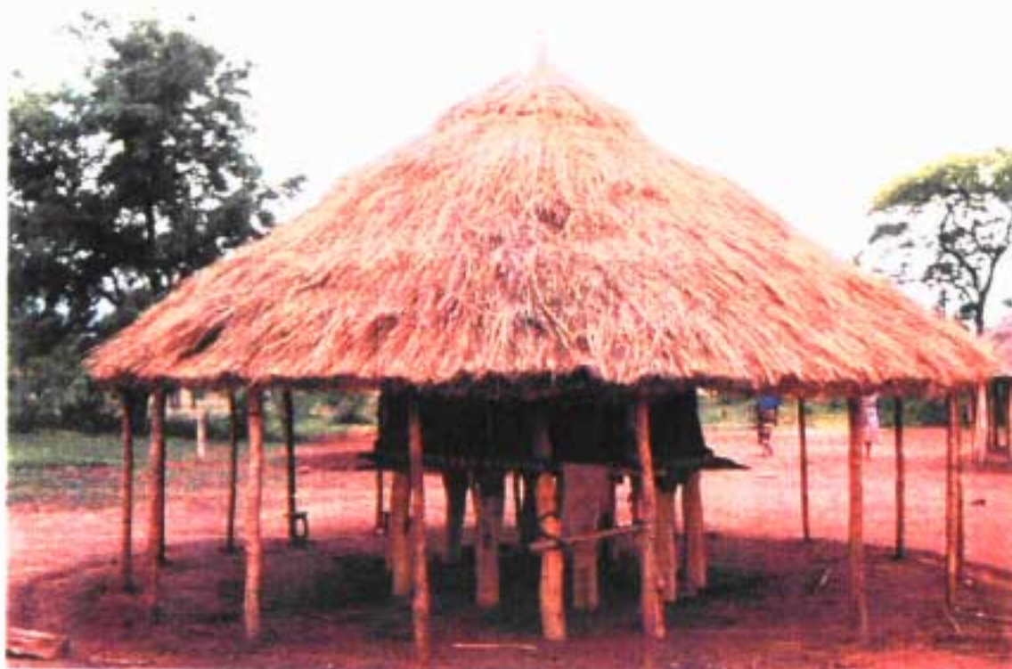
Plate xi. Mola farmer's modified store - 1; note the use of more slender than normal vertical posts to support the roof (see page 16)
