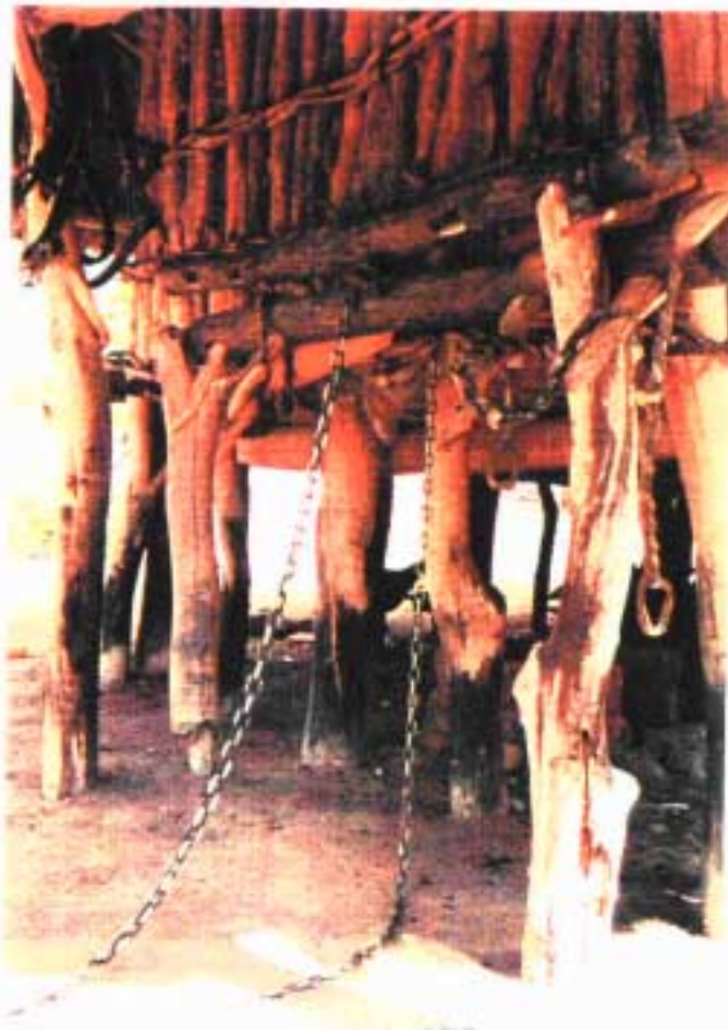
Plate xix. Posts treated with old engine oil; note also damaged posts (see page 22) (timbers with chains are yokes for oxen)
