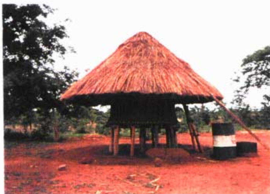
Plate xii. Mola farmer's modified store - 2; note the absence posts to support the roof which rests entirely on the wall of the store (see page 16)
