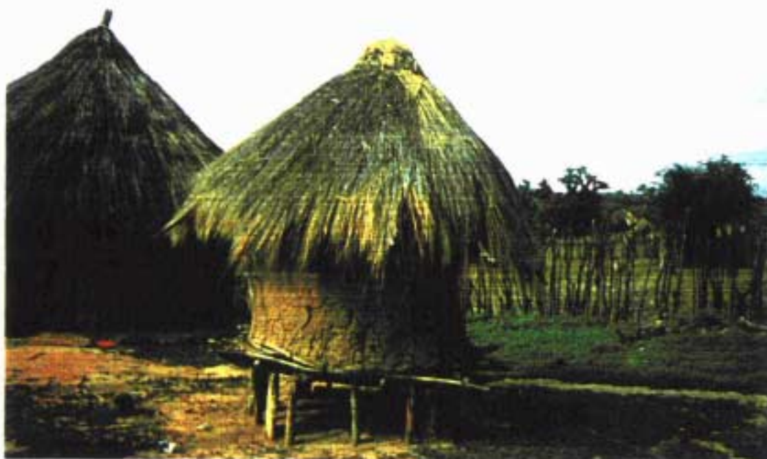
Plate xxvi. Cracked mud walls harbour infestation which is difficult to eradicate (see page 35)
