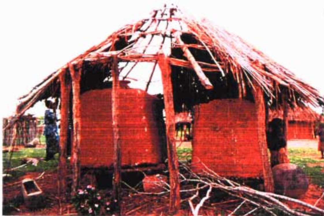
Plate xxiv. Poorly maintained store; note the poor hygiene with bird droppings around the top of the left-hand container (see page 35)
