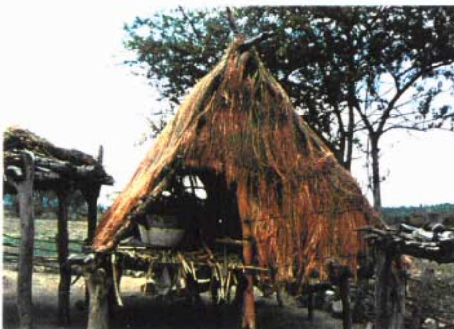
Plate xvi. Triangular shaped shelter on drying platform (Dumba); shelter built using crop residue and poles (see page 18)
