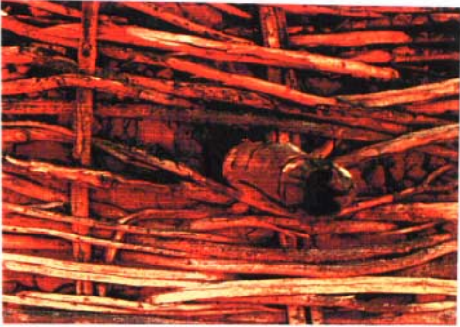
Plate xxii. Pole running through a store to form a step externally and internally; note the gap around the pole providing access for pests and vermin (see page 34)
