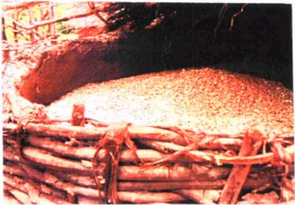
Plate vii. Basket store showing internal plastering (see page 8)
