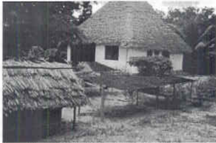
Domestic PV Installation, Near Malindi, Kenya
