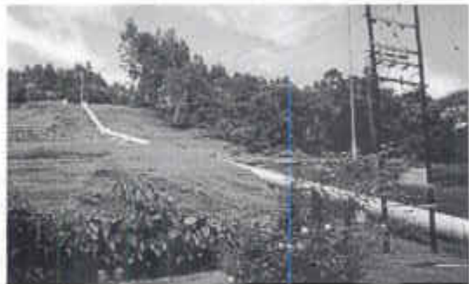
Tea Estate Hydro Installation, Near Kericho, Kenya
