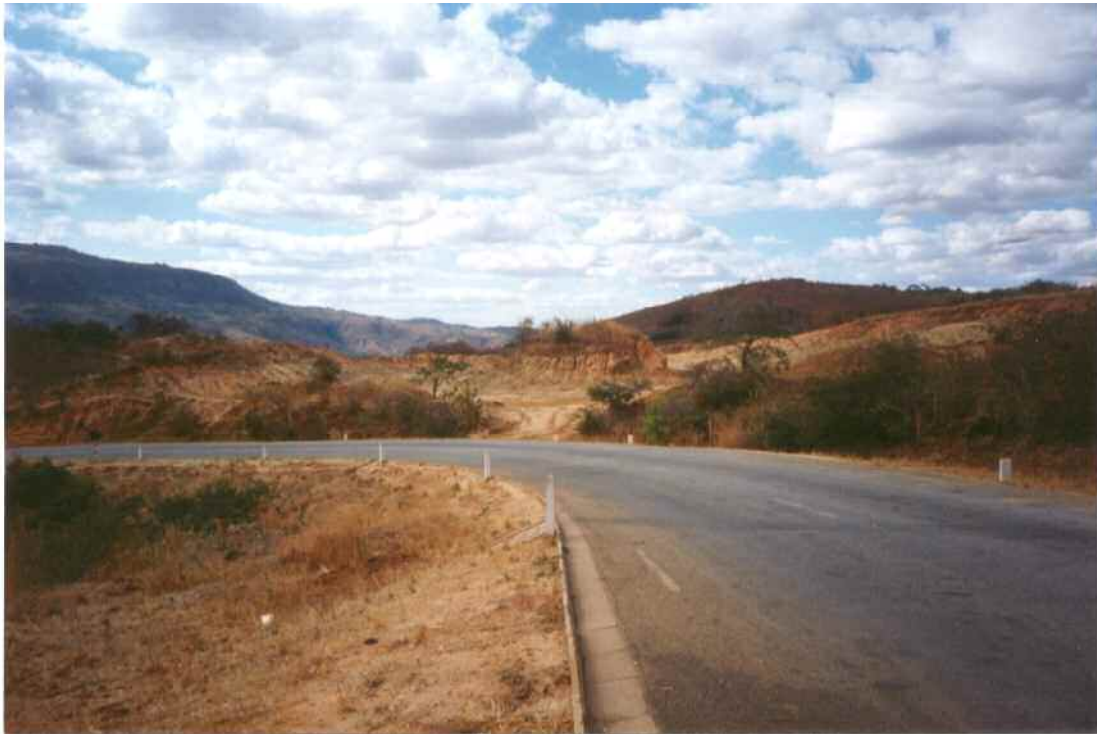
Plate 4-1 Un-reinstated borrow area in an area of natural beauty; Zimbabwe
