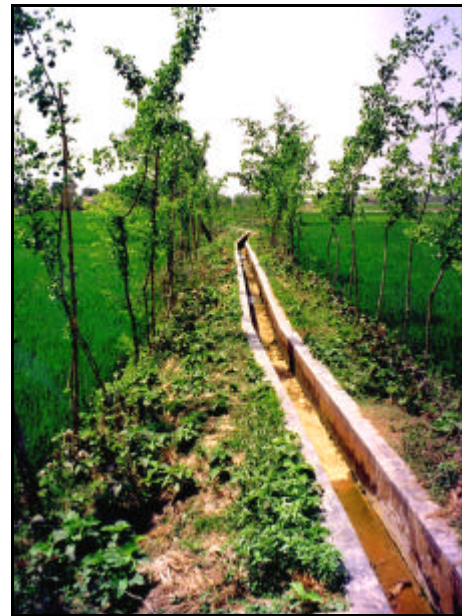
Lined earth channel
