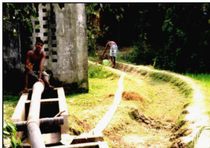
Surface pipe system
