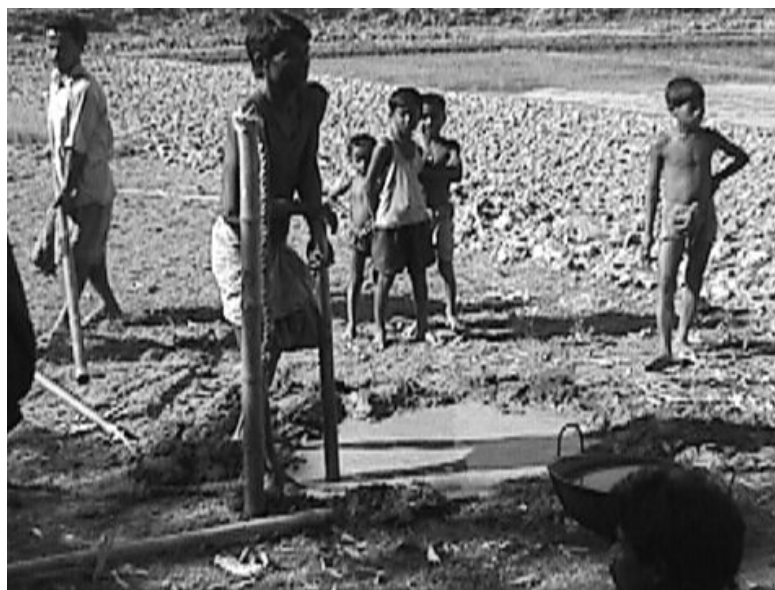
Figure 4: Mistry Starting a Hole with 1.5m Pipe
