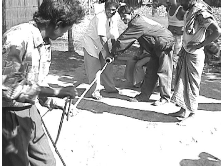
Figure 17: Cleaning the Pith out of the Bamboo
