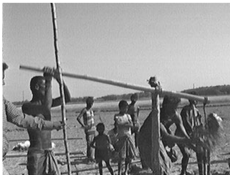
Figure 1: Mistries Operating Sludging Equipment
