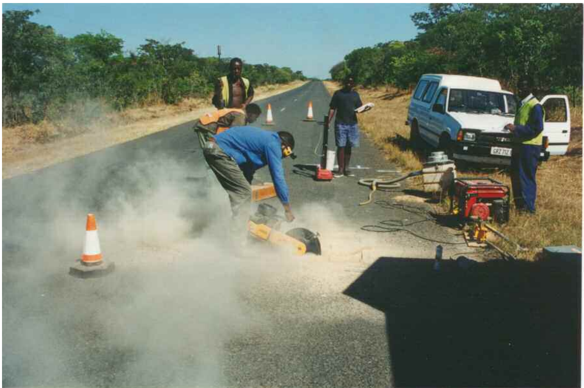
Plate 4-1 Hand saw used to cut stabilised roadbase
