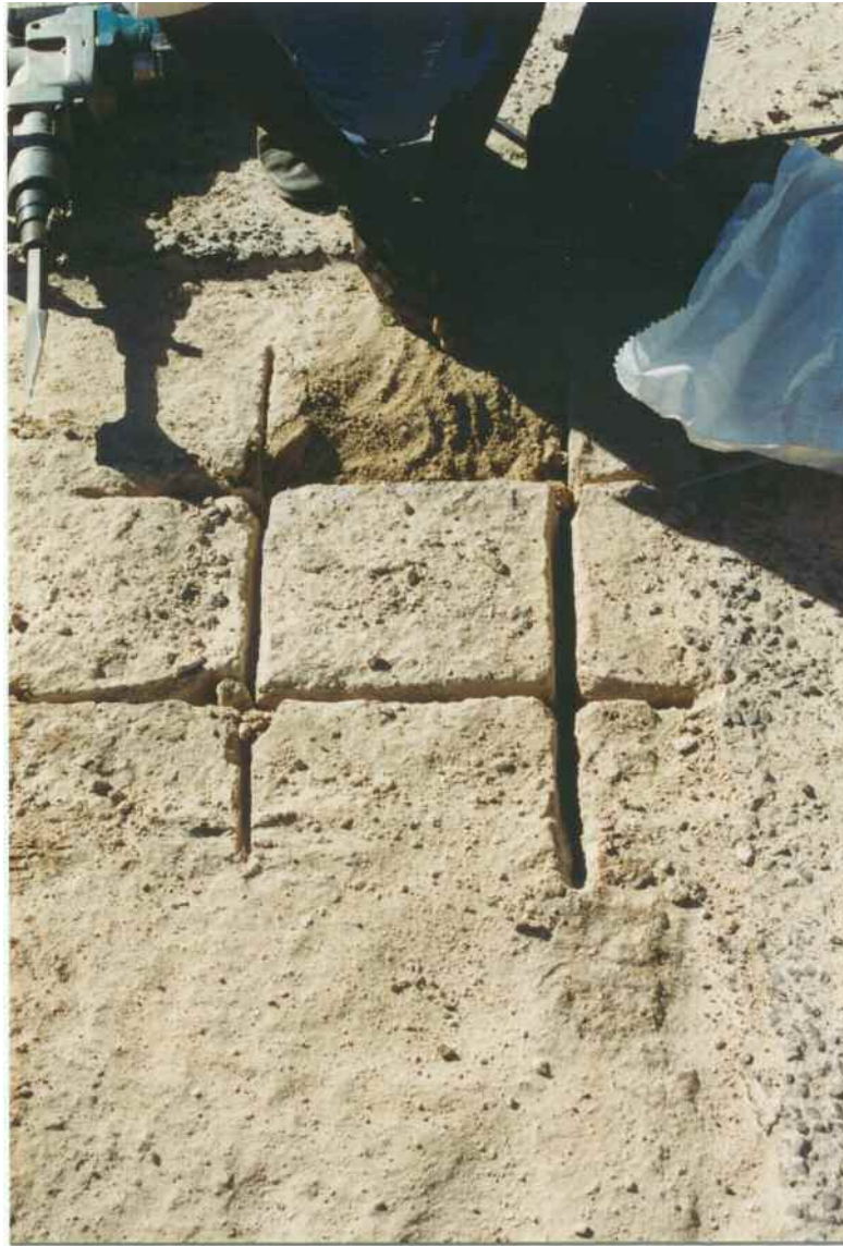
Plate 4-2 Blocks of roadbase lifted from road for laboratory testing
