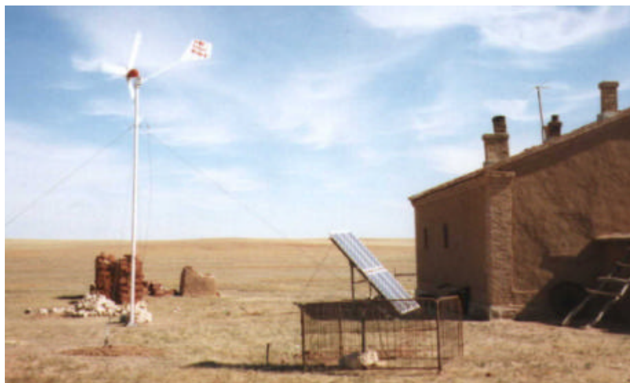
Figure 23 Wind/PV Hybrid Demonstration System
