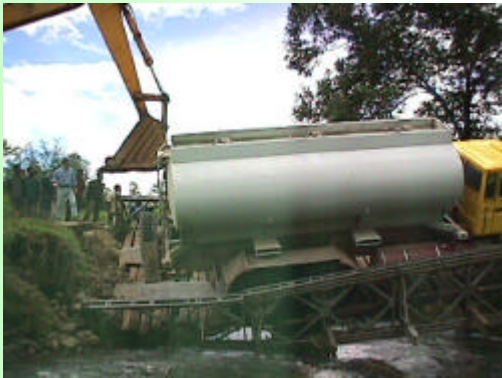
A lorry too heavy for the poorly maintained bridge.
