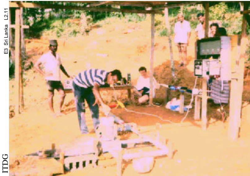
Installation of hydro system in Sri Lanka
