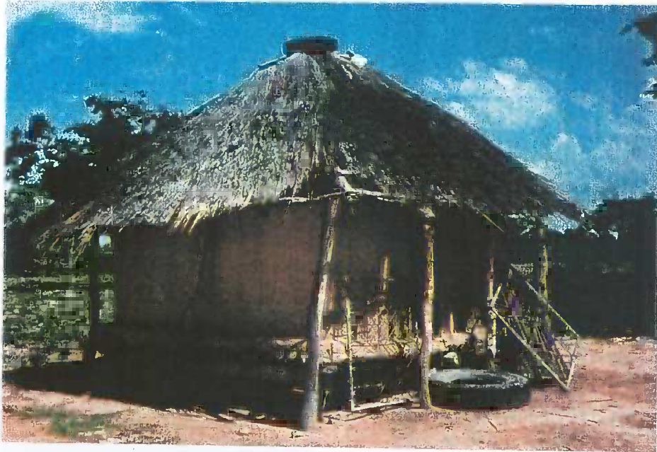
Figure A1.1 Rectangular grain store on a raised platform
