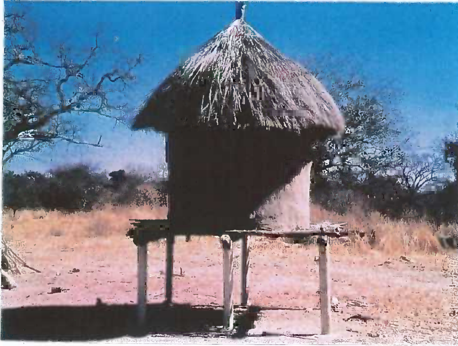
Figure A1.5 Modified timber-based store incorporating PVC plastic legs filled with concrete
