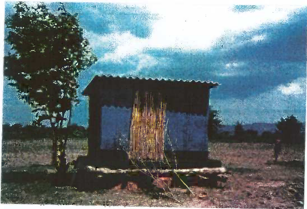
Figure A1.4 Brick-built rectangular store
