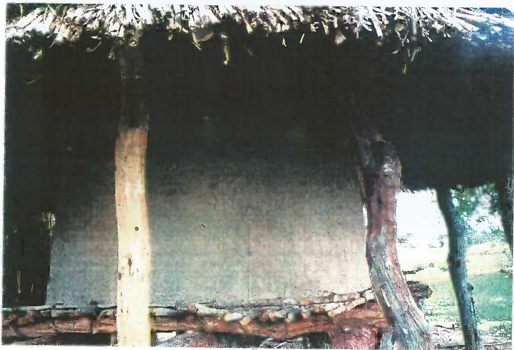
Figure A1.2 'Bottle-shaped' grain store on a raised platform
