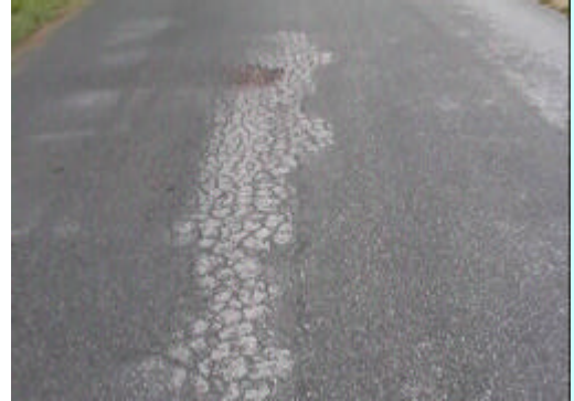
Severely Cracked Surface
