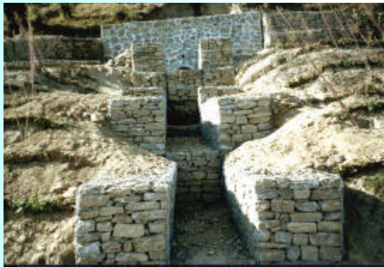
Cascading Gabions preventing Soil Erosion
