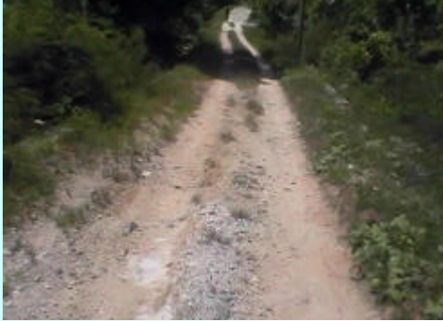
Poor Quality Gravel Road – Track
