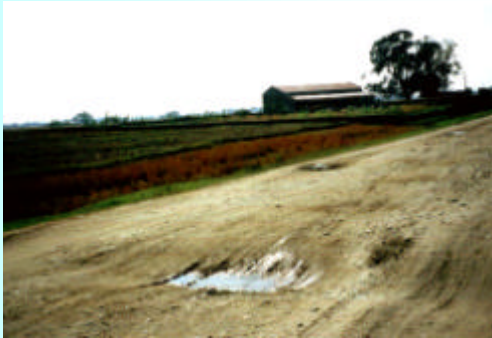
Pothole collecting Water on a Gravel Road
