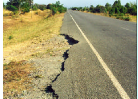
Poor Shoulder Maintenance
