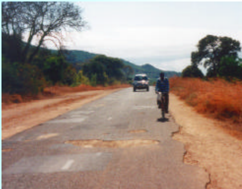
Paved Road in a Poor Condition
