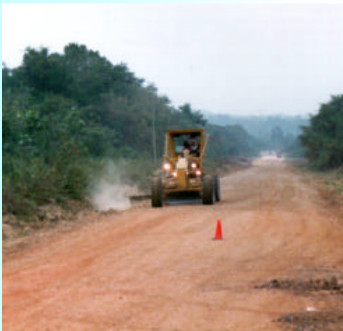
Regular Grading of Gravel Roads
