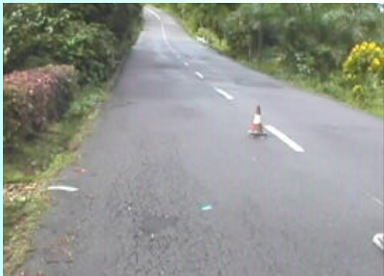
Crocodile Cracking Failure
