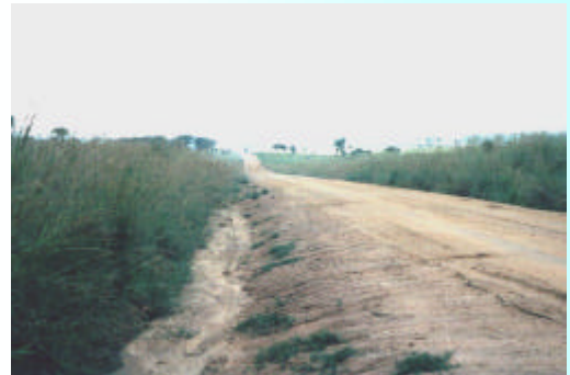
Silting Side Drains
