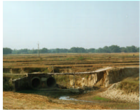
Culvert Failure with Poor Repairs
