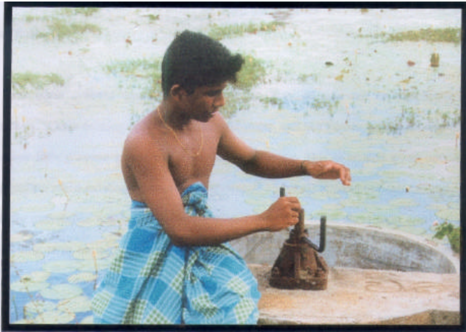
Photograph: 4 H M Nishankau is working on his father's paddy. The sluice gate is opened to release water into irrigation channels. The "key" is allocated to specific members according to a pre arranged schedule.
