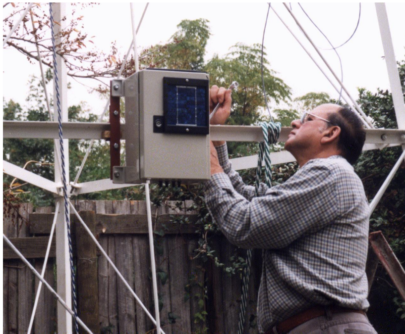
Figure 3.8: Installing the monitoring system in South Africa
