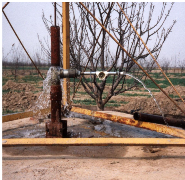
Figure 3.7: Problem of leakage out of the well head riser
