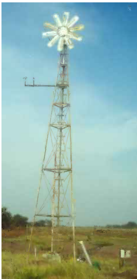
Figure 3.2: IT Power windpump in India
