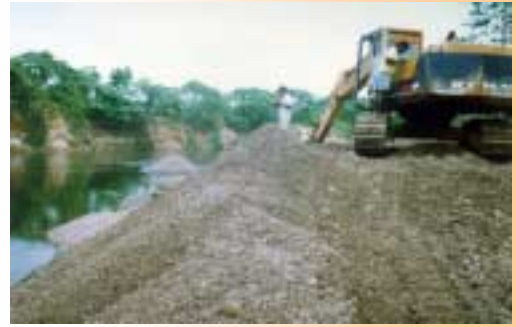
Try to use the same plant to excavate and load aggregate
