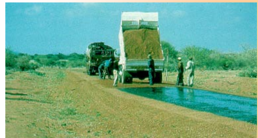
When stabilisation is necessary consideration should be given to the economics of extending the life of the road surface by the application of a low cost bitumen seal, such as an "otta seal" (as shown above) or a sand seal. (Photograph courtesy of Botswana Roads Department).
