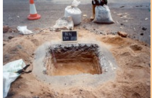
Pavement trial pit exposing construction materials in a lightly trafficked bitumen surfaced road
