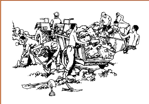
Manual methods of site clearance are encouraged, because they reduce damage to fragile topsoil and subsoil materials (Sketch after ILO/ASIST Bulletin No 9, 1999)
