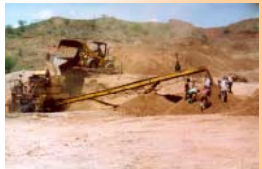
Mobile screening plant producing road material. Note team of men flattening the stockpile and reducing segregation
