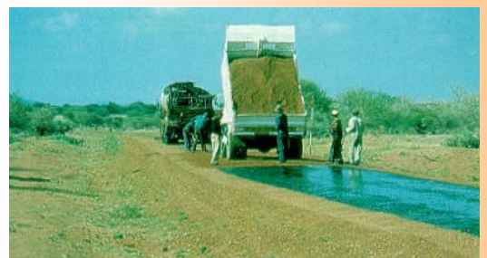
"Otta" Seal under Construction (photo courtesy of Botswana Roads Department)
