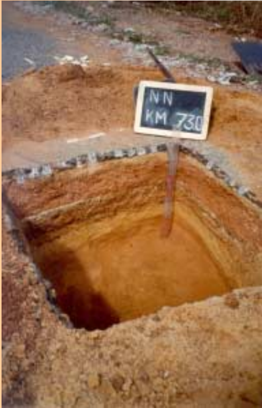
Paved road built with “as dug” laterite and sand.
