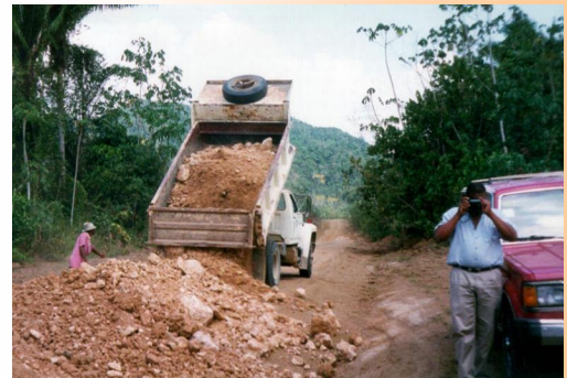
High proportion of oversize being supplied to the road
