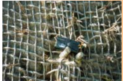
Placing jute nets in preparation for grass planting
