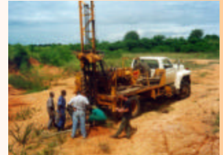
Borrow Pit Site Investigation
