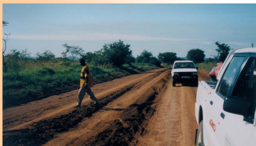
Material with too much plastic fines producing a slippery dangerous surface.
