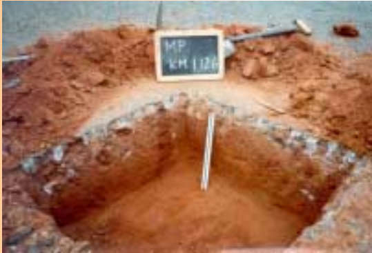
Pavement trial pit exposing lower standard, but satisfactory, natural gravel construction materials.
