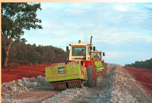
Grid roller treating oversized material on the road (Photos courtesy of Broons Hire (SA) Pty Ltd)
