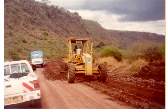
The binder content of wearing course gravels may be improved during regrading by bringing some plastic subgrade soil from the side of the road.
