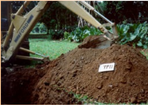
In each trial pit all layers should be accurately described and measured. Materials proposed for use should be sampled and tested.
