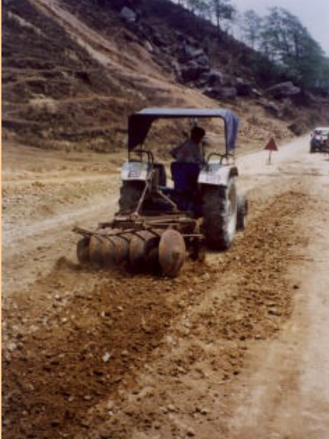
Disc harrow being used to prepare ground for treatment
