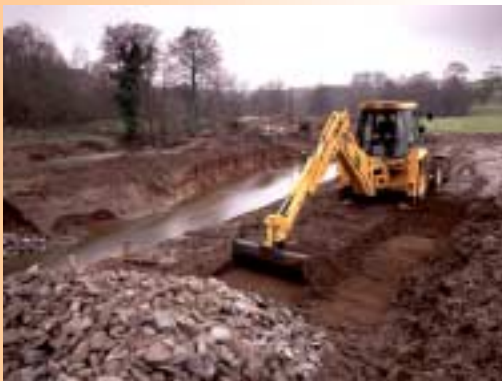
Tractor excavator carrying out top-soil stripping (photo courtesy of JCB)
