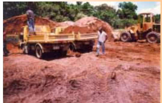
The pit stockpile areas should be maintained so as to allow easy movement of haulage vehicles
