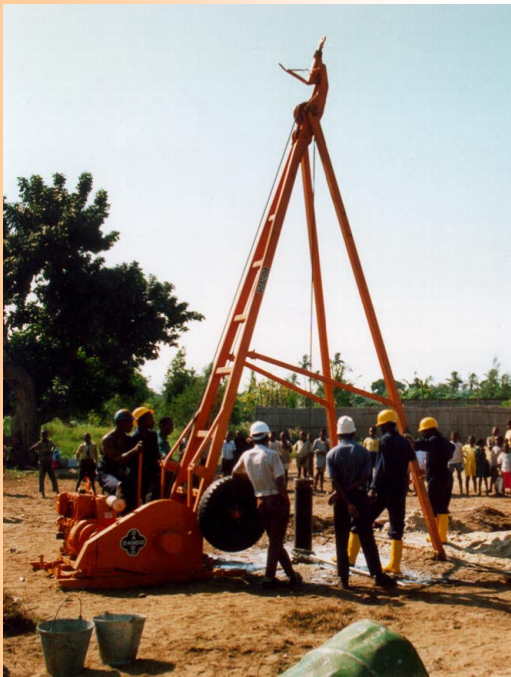
Cable tool boring rig, Dando 3000 Buffalo Rig shown. (Photo courtesy of Dando Drilling International)
