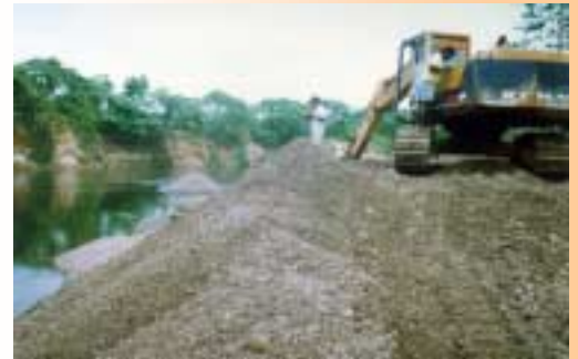
Excavator digging river gravel from below water level
