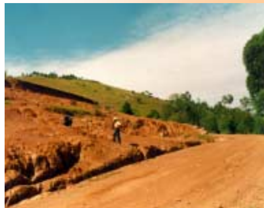
Pits should not be developed adjacent to the road when it can be avoided.
