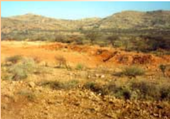
Extraction of thin near surface gravel involves disturbing a large area of land for a relatively small quantity of road material. Careful reinstatement should be carried out as an area of the pit is worked out.
