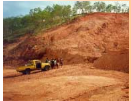
Do not forget the need to repair damage caused by excavation. In some cases associated costs will be significant.
