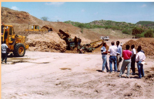
Small mobile screening plant producing gravel wearing course
