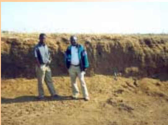
Extraction of thin near surface gravel involves disturbing a large area of land for a relatively small quantity of road material. Careful reinstatement should be carried out as an area of the pit is worked out.
