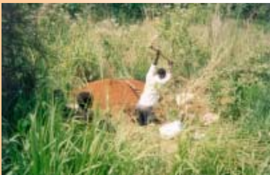
Manual trial pitting during a materials search
