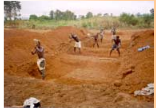
Labour based gravel pit development (Photo courtesy of P Larcher, Univ. of Loughborough)
