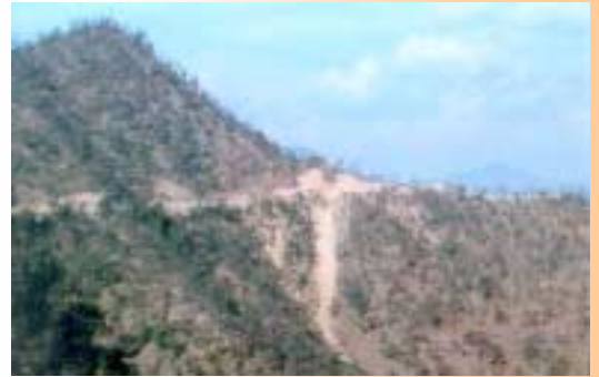
Side tipping of overburden in mountainous terrain is unsightly and frequently leads to severe slope instability problems.
