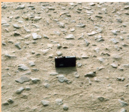
Dusty rough surface containing oversize and not enough plastic binder material
