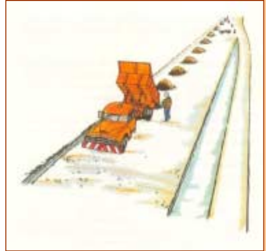
Material supply for regraveling (Sketch from PIARC International Road Maintenance Handbook, 1994)
