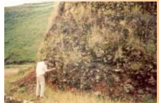
Rippable volcanic scoria gravel in road cutting.
