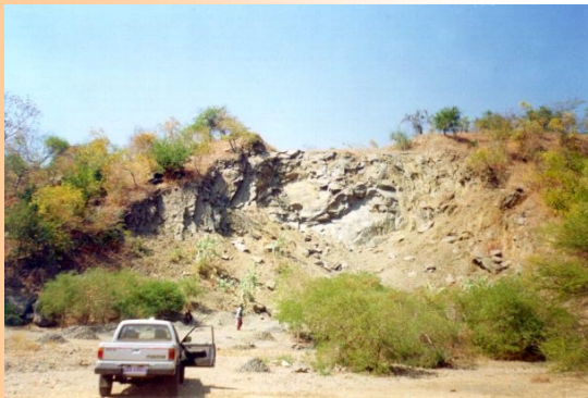
A field survey to collect “up to date” borrow pit information and verify existing records should, if possible, accompany the establishment of a Materials Resource Database. This survey should involve completion of a specially designed “Field Proforma” that will ensure collection of all required field information in a format that will allow easy entry onto the database via a “Data Entry Proforma”.
