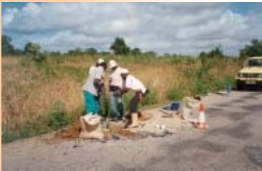
Investigating construction materials in a low volume paved road.
