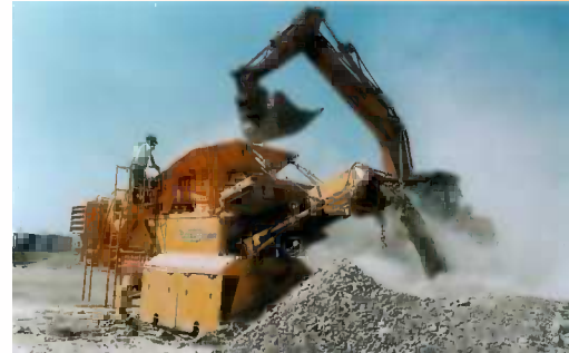
Mobile Crushing Plant in operation (Photo courtesy of Pegson).
