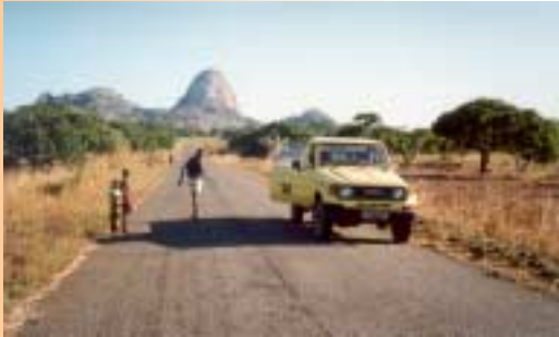
Typical lightly trafficked bitumen surfaced rural road.
