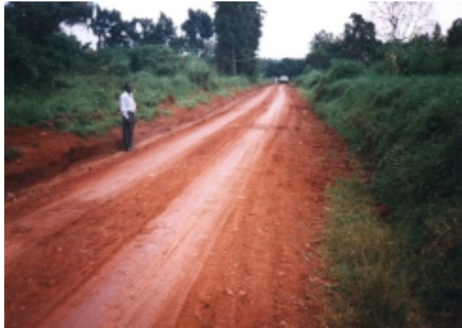
Photograph 3-1 Section of Road Prior to Treatment
