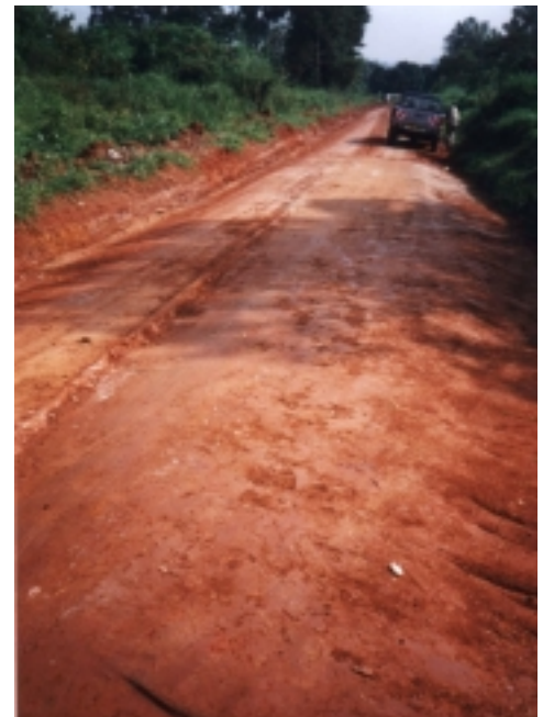
Photograph 3-3 Completed Control Section Comprising Laterite Only
