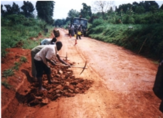
Photograph 3-2 Method of Excavation
