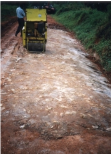
Photograph 3-6 Compaction
