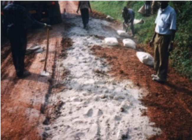
Photograph 3-5 Methods of Adding Lime
