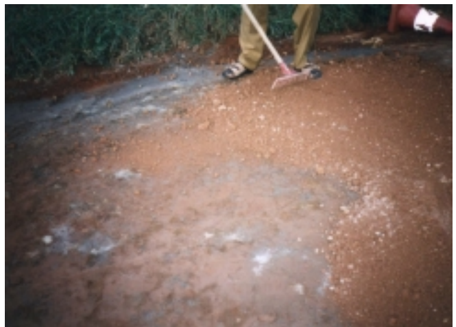
Photograph 3-7 Application of Sacrificial Layer
