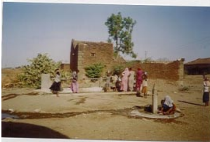
7. Stand post with taps installed by the project as an entry point activity.
