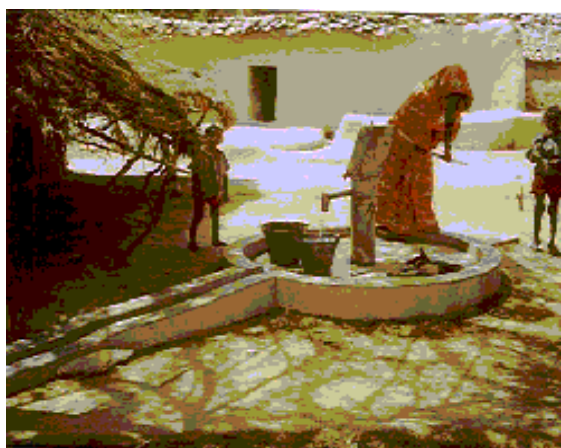
8. Bore well with hand pump installed through the project as seen in Nayapurva village.
