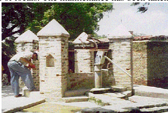
3. Hand pump installed on the dug well, which reduces the strain on women to pull water
