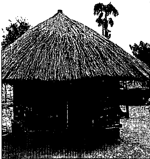
Fig. 2. The experimental store (composed of 6 bins) used in Binga district and Harare.
