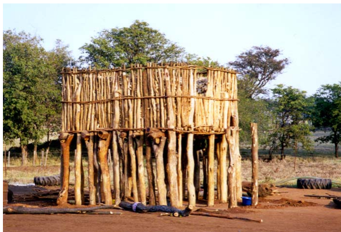
Plate 2.5.2 Nturuka granary under construction, Mahlathi, Lowveld District
