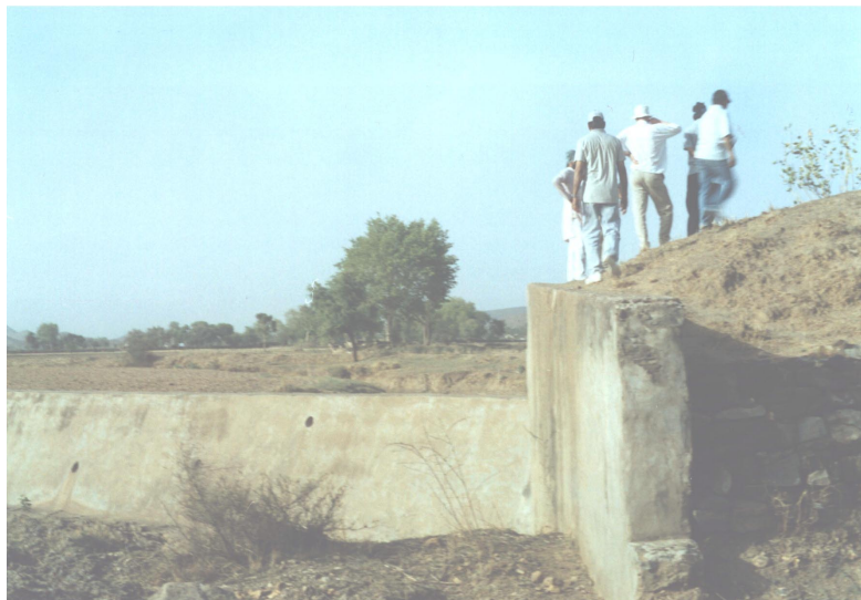
Plate 2 Typical spillway structure on a bundied field, Alwar District, Rajasthan, India.
