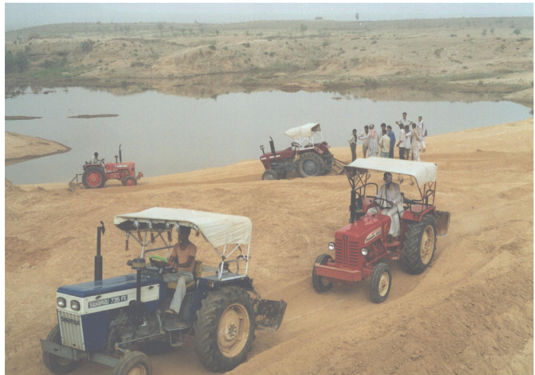
Plate 1 Construction of an earth dam by a community of farmers in the Alwar district, Rajasthan, India.
