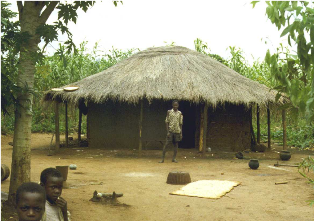
Figure 4. A typical household structure found in Zambézia Province. The main difference found in some areas is the use of palm leaves for roof thatching. Typically, up to seven or eight people may sleep inside. Food is stored in the same structure on a raised platform within. The cooking fire is often below the platform, providing smoke which is used to reduce insect infestation. Farmers estimate an average of 50 rats live in the roof thatching at any given time.
