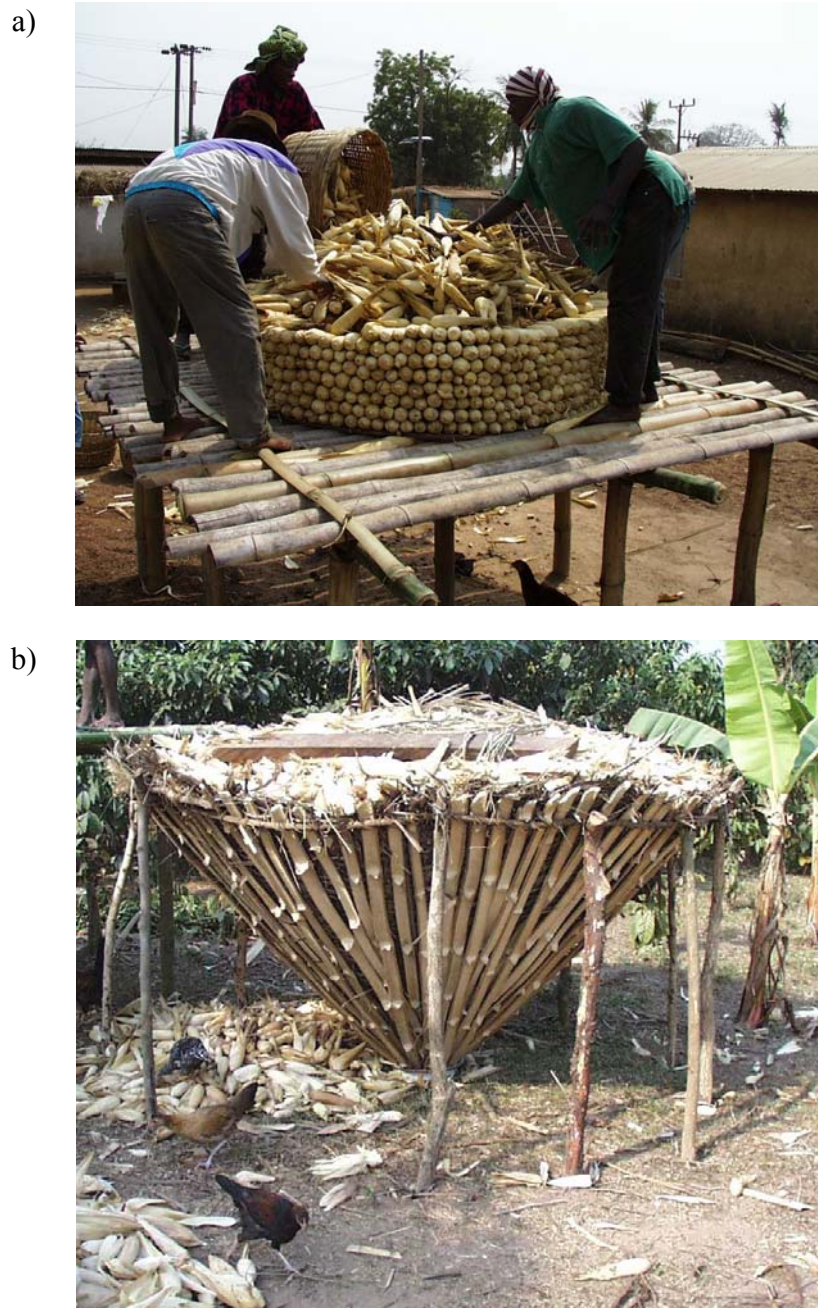
Figure 4.1: Two common structures for the storage of maize cobs in the Volta Region of Ghana, a) an Ewe-style barn under construction, which has an thatched roof added at the end and b) an inverted cone
