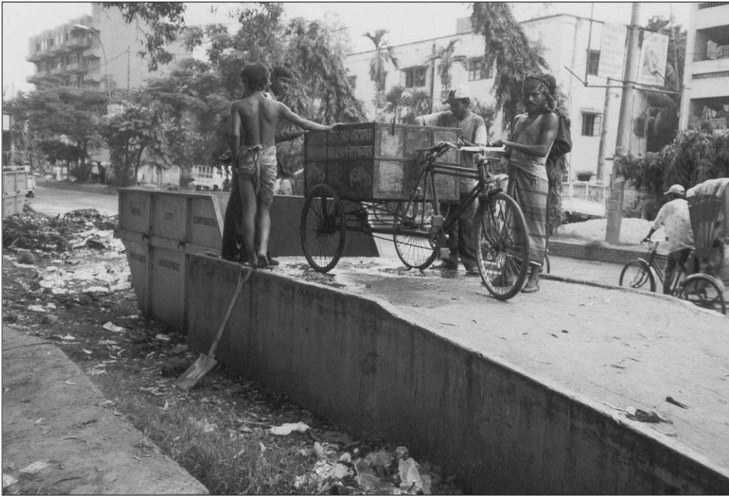
Ramp transfer system in Khulna, Bangladesh
