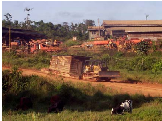
BCL transporting field accommodation to new site
