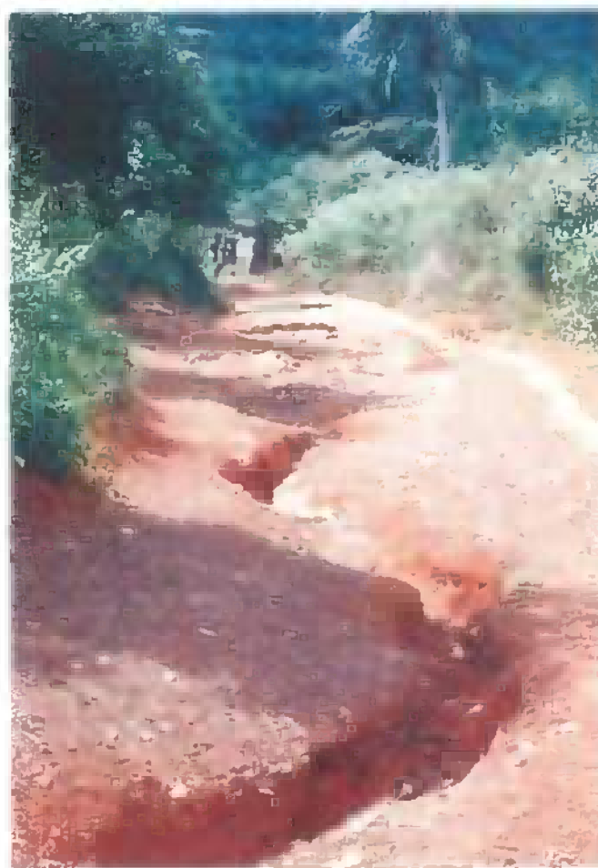
Figure 18. Gully development at the start of path 1, the route to the River Okye (Sampa village)
