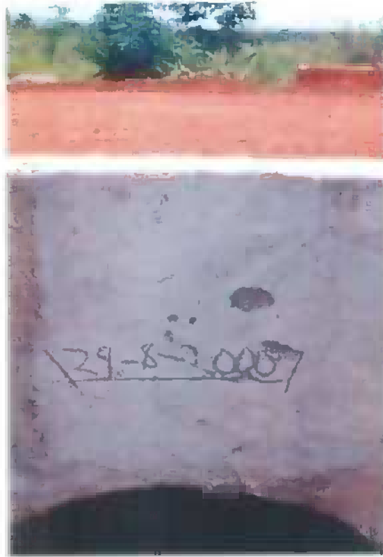
Figure 11. A road culvert along the new Abora-Ankamu feeder road
