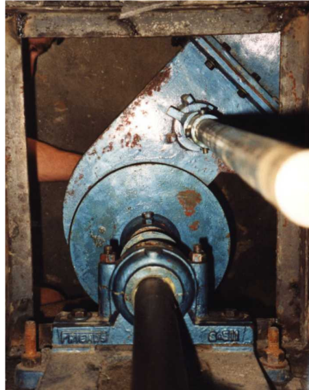
Crossflow assembly from inside the mill-house
