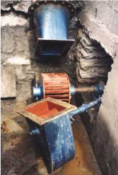
Assembly of nozzle, valve and runner
