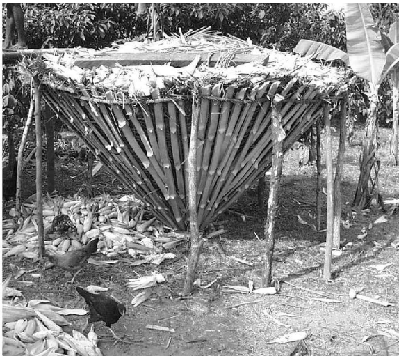
Figure 1. Two common structures for the storage of maize cobs in the Volta Region of Ghana, a) an Ewe-style barn under construction, which has an thatched roof added at the end and b) an inverted cone.
