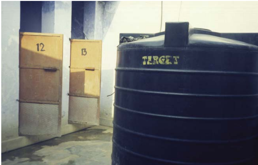
Figure 21 The water storage tanks at the Rahul Gandhi Camp Sulabh block need to be filled every three days and ensure a regular supply of water, if water use is controlled.
