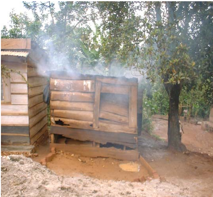
Figure 6: A kitchen with poor ventilation and poor air circulation. There is a likelihood of indoor exposure to smoke.
