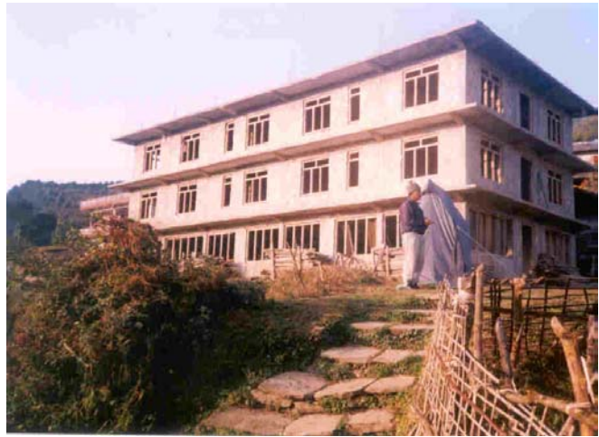
Figure 17: New hotel under construction in Ghandruk
