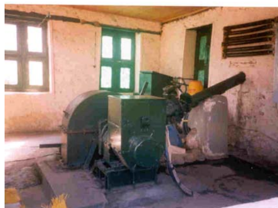
Figure 16: Interior of Ghandruk power house
