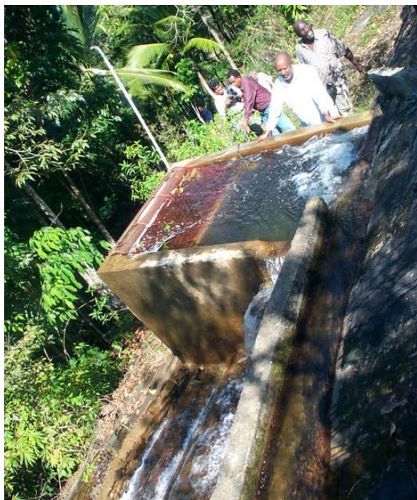
Figure 19: An example of a penstock at the source of the hydro intake. In Hettikanda and Handunella, this was built by the community
