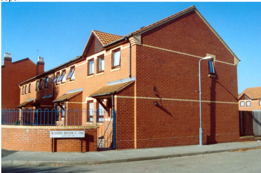
Figure 6. Housing Association accommodation for Bangladeshi widows in Birmingham.
