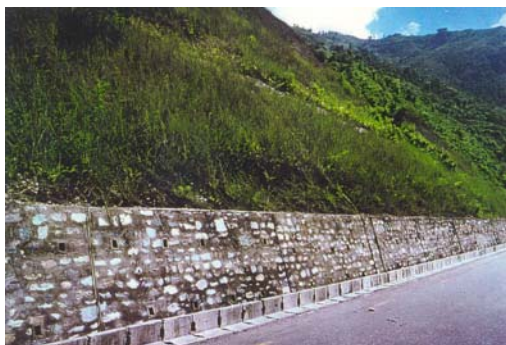
Bio-engineered surface erosion protection with masonry toe wall
