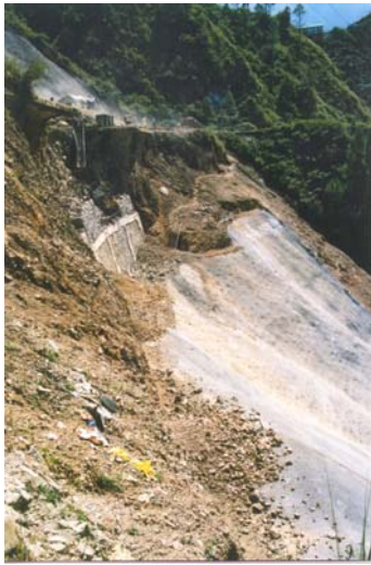
Shotcrete surface erosion protection
