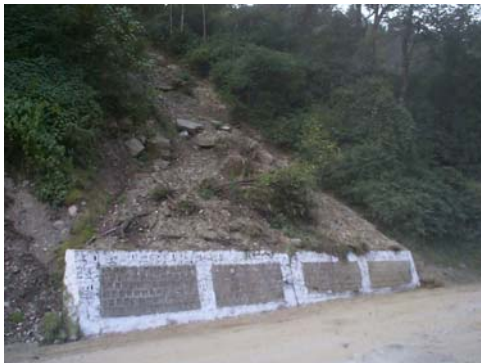
Mortared masonry retaining wall to retain loose granular colluvium
