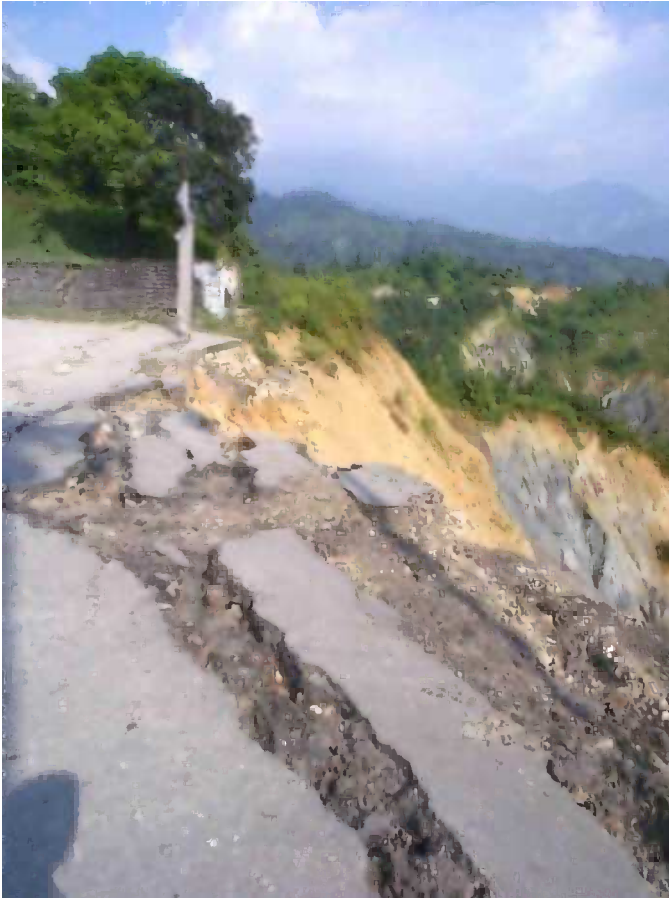
Severe cracking to road, as a result of undercutting by a landslide.
