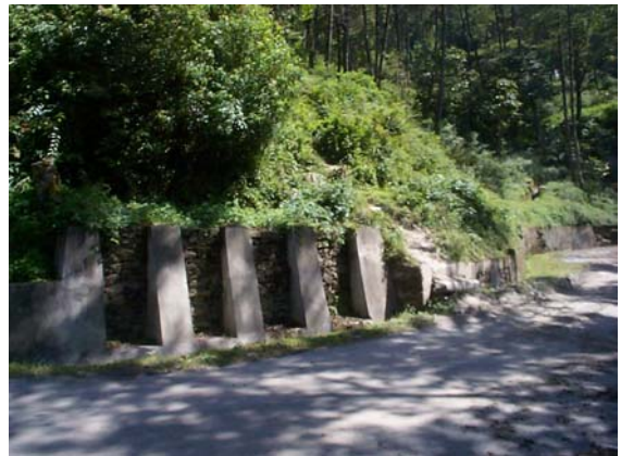
Mortared masonry retaining wall with mass concrete ribs for support
