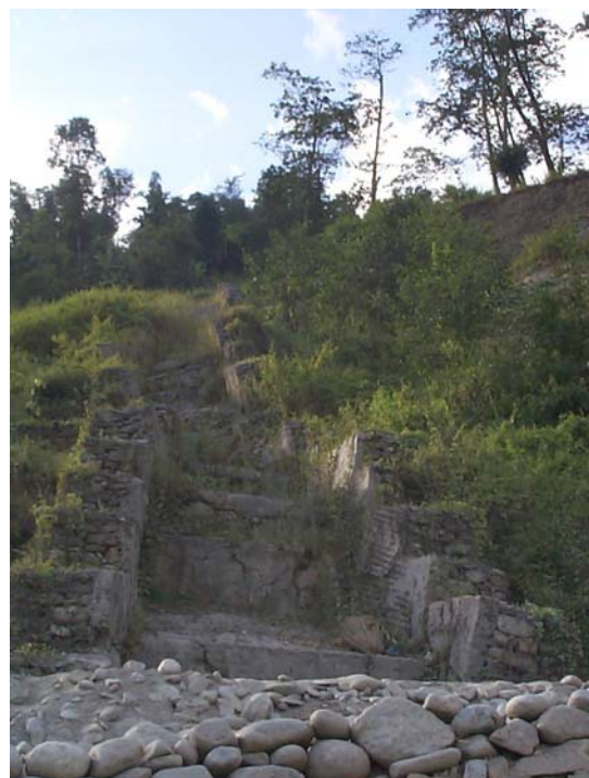
Damaged gabion cascade channel located on a slow moving landslide
