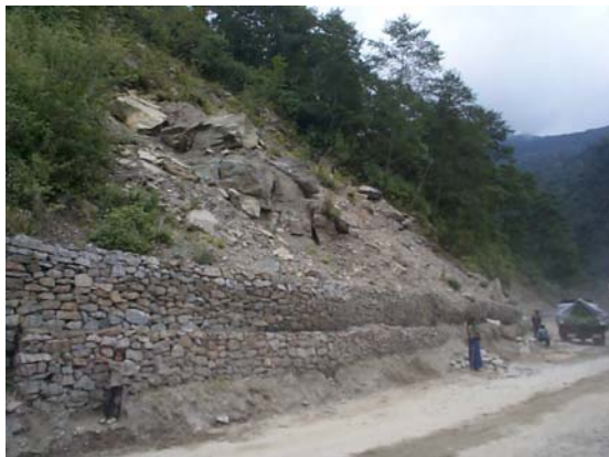
Gabion toe wall used to stabilise a shallow landslide (though poorly constructed)
