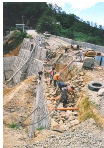
Reinforced concrete composite walls with mortared masonry infill panels
