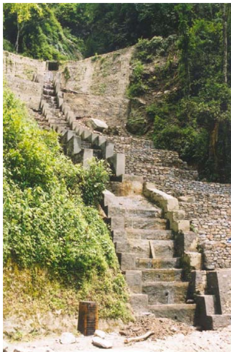
Masonry cascade channel constructed on a relatively stable slope.
