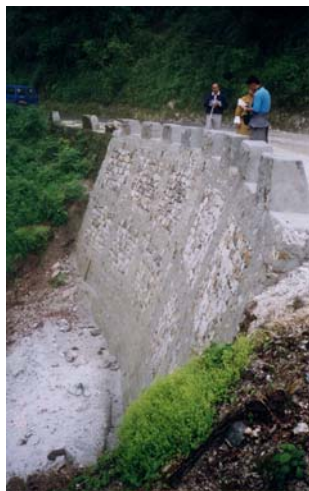
Reinforced concrete composite walls with mortared masonry infill panels
