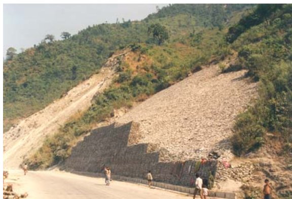
Gabion toe wall with hand placed rock backfill for stability and surface protection
