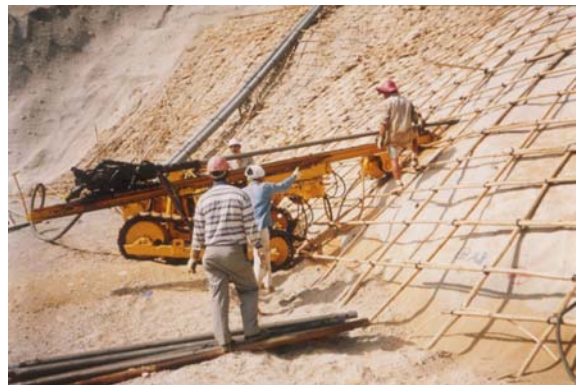
Installing soil nails
