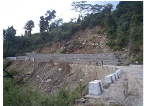
Gabion retaining wall to support a shallow failure in colluvium
