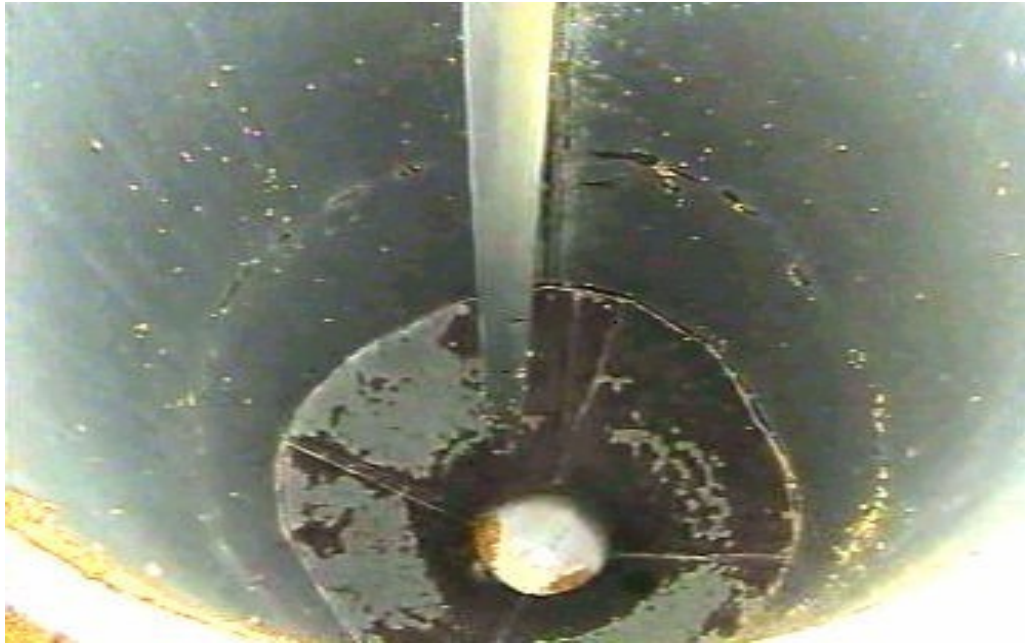
Empty bin with the Perforated Steam Pipe
