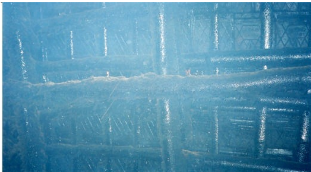
Plate 7.3 Rafters in the Kitchen covered with Tar.
