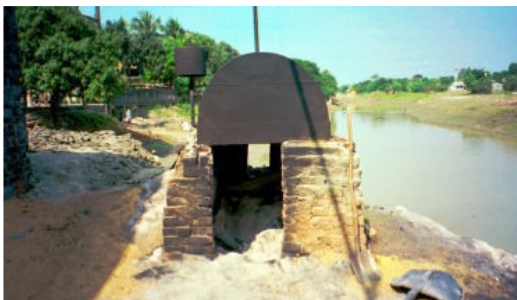
Plate 2.1 Semi Cylindrical Boiler with an Open Furnace
