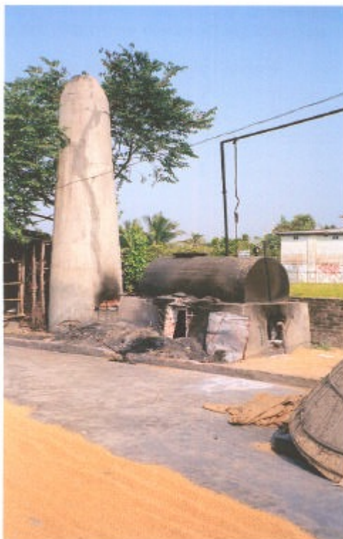
Plate 2.2 Cylindrical Boiler with Poorly Constructed Furnace
