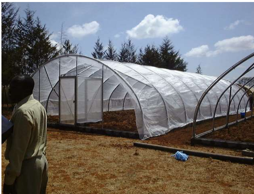
Figure 1.3.1 Construction of screenhouses at Thika, NARL
