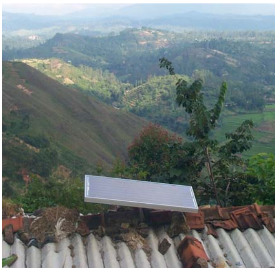
Photovoltaic panel on roof of a private home
